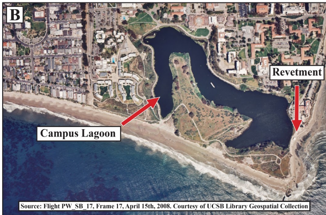
Figure 22: Aerial photograph of Campus Lagoon region from (A) 1928 and (B) 2008. In 1942, a revetment consisting of beach sand and cobbles was constructed across the opening of the southeast region of the lagoon, preventing tidal influence (Jones & Stokes Associates, Inc., 1999). Water levels within the lagoon are sustained by the discharge of seawater by operations related to UCSB Marine Science research (Jones & Stokes Associates, Inc., 1999).
