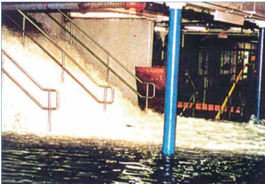
Subway flooding in New York during a 1992 Nor'easter
