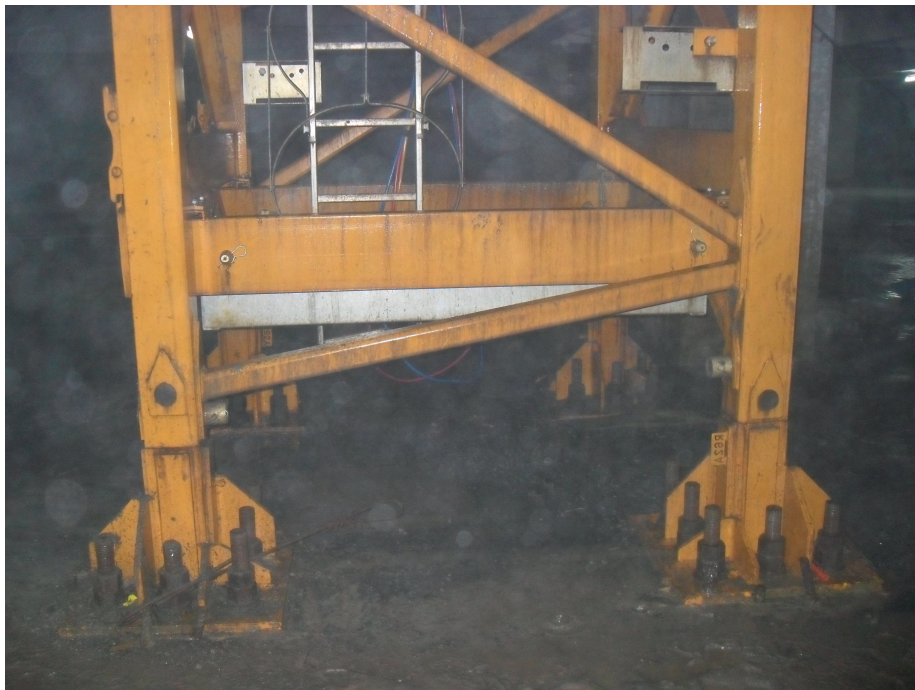
Figure 11: Tower Crane Foundation
