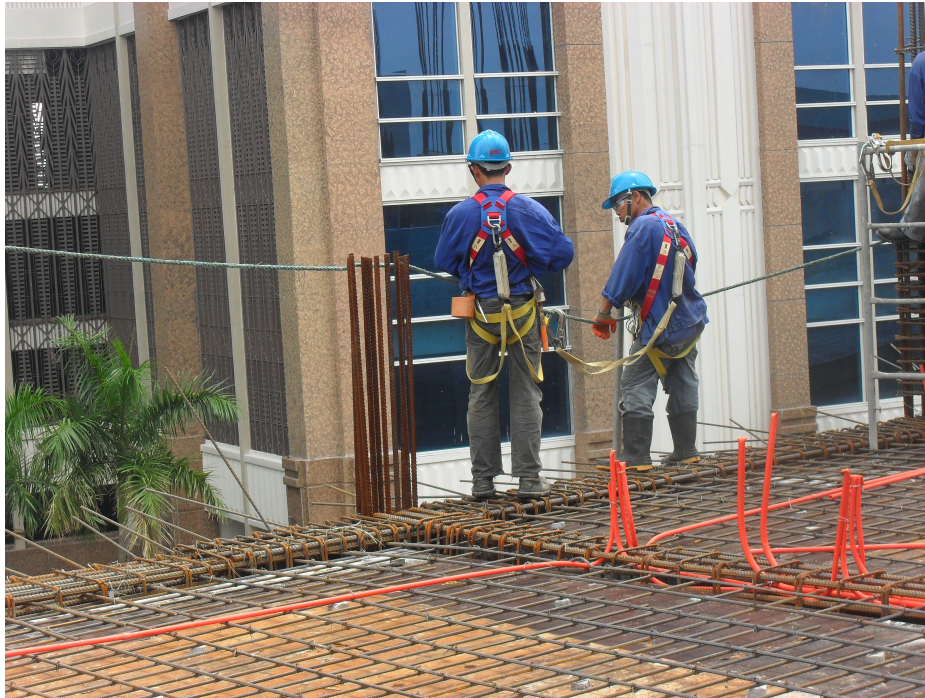
Figure 10: Fall Protection System
