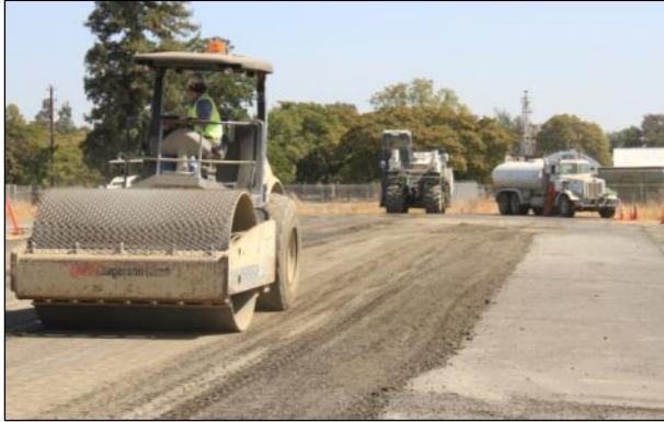
Figure 3.10: FDR-NS: Compaction with smooth drum roller.
