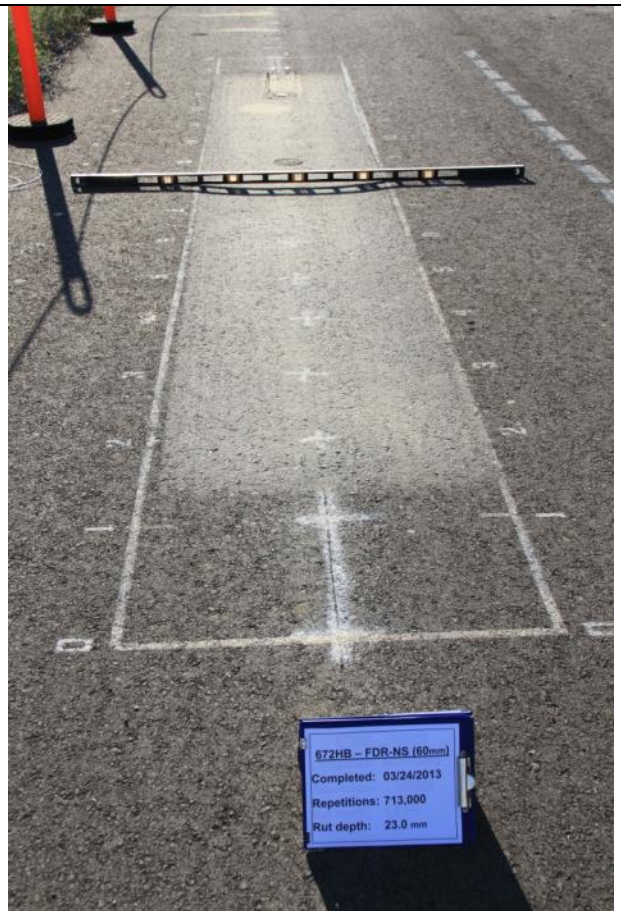
General view of test section looking from west to east
