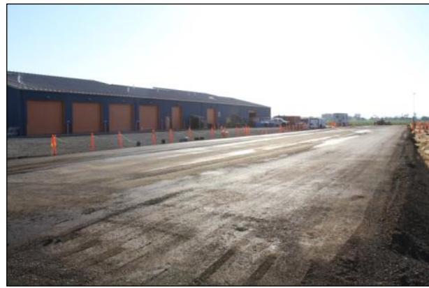
Figure 3.11: FDR-NS: Surface leveling with a grader.
