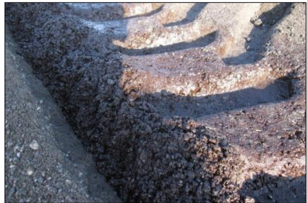
Figure 3.15: FDR-EE: Inconsistent emulsion application across width of test track.
