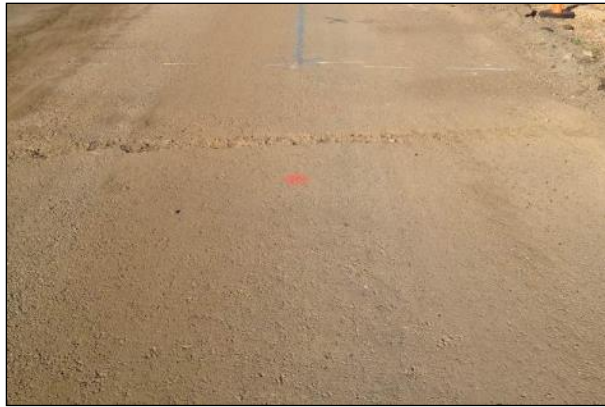
Figure 3.34: Broomed surface of FDR-NS layer.
