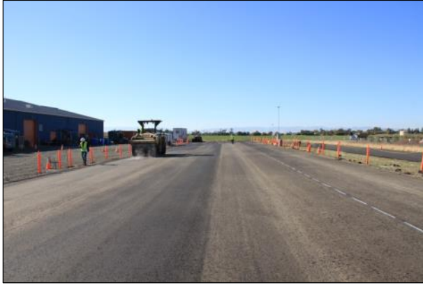
Figure 3.38: First lift of asphalt concrete after compaction.
