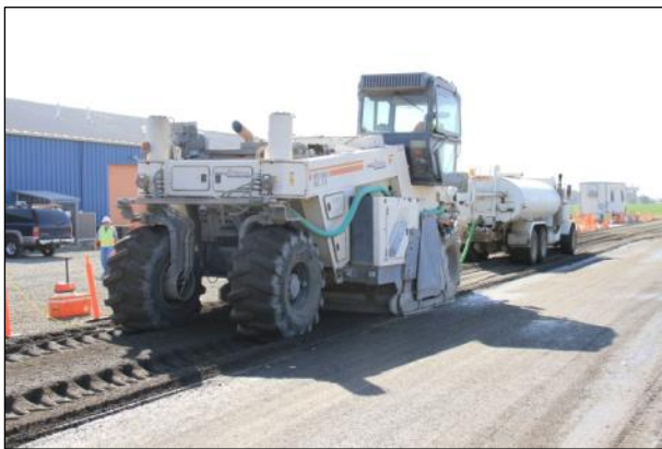
Figure 3.29: FDR-PC: Uniform mixing after first pulverization pass with no water.
