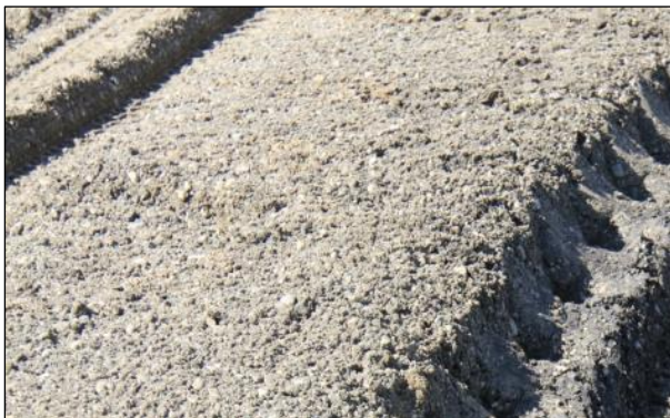
Figure 3.8: FDR-NS: Pulverized material.
