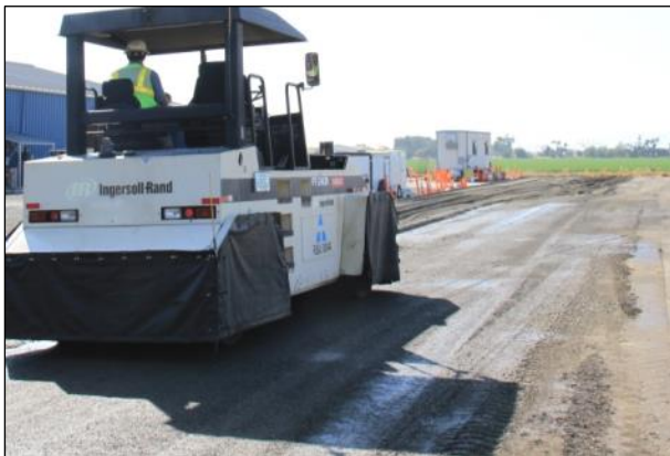
Figure 3.12: FDR-NS: Compaction with rubber-tired roller.
