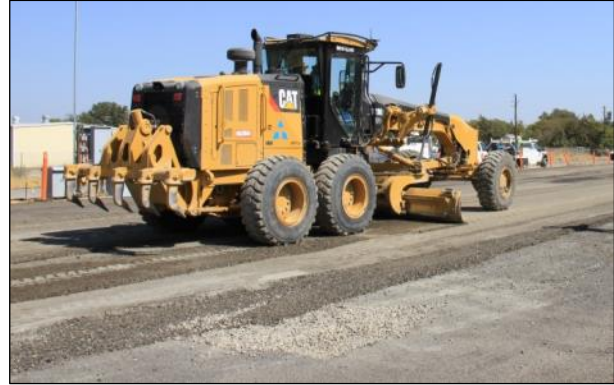
Figure 3.11: FDR-NS: Surface leveling with a grader.
