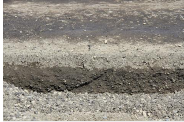
Figure 3.20: FDR-EE: Excavation showing wet recycled layer.
