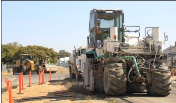
Figure 3.5: FDR-NS: Test track recycling.
