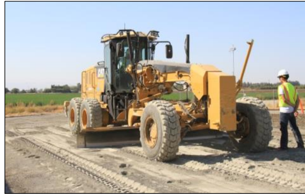
Figure 3.28: FDR-PC: Removing excess cement on Cell #8.
