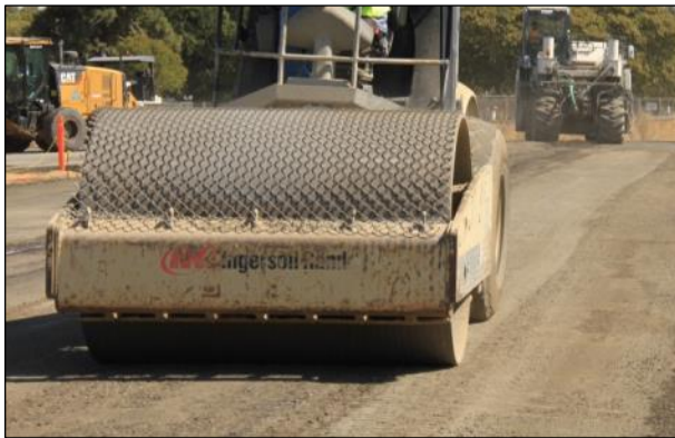
Figure 3.23: FDR-FA: Uniform mix behind recycler.
