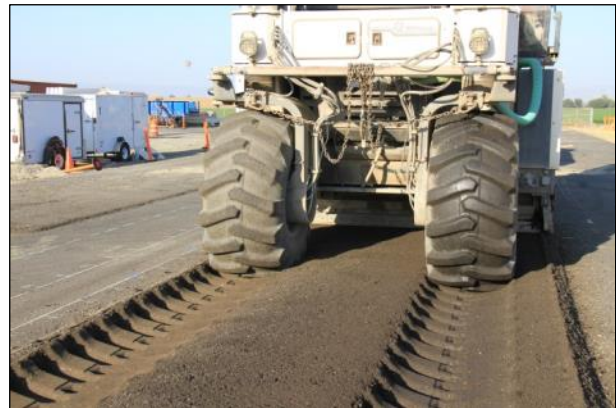
Figure 3.15: FDR-EE: Inconsistent emulsion application across width of test track.
