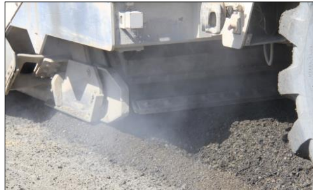
Figure 3.5: FDR-NS: Test track recycling.
