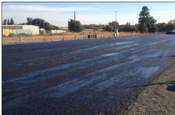
Figure 3.36: Prime coat application.
