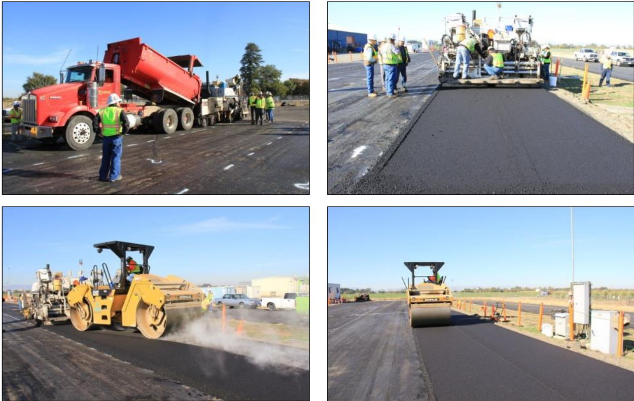
Figure 3.37: Asphalt concrete placement.
