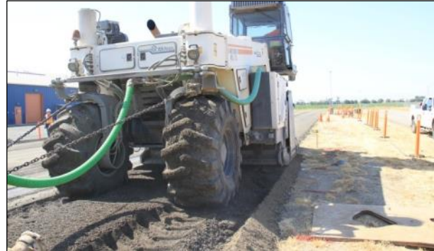
Figure 3.5: FDR-NS: Test track recycling.
