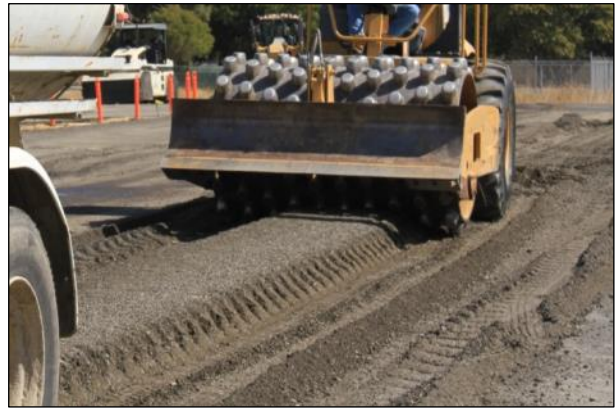
Figure 3.24: FDR-FA: Padfoot roller compaction on uniform mix.
