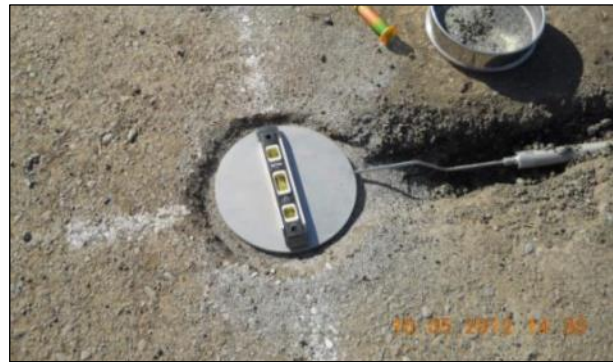
Figure 4.4: Pressure cell installation.
