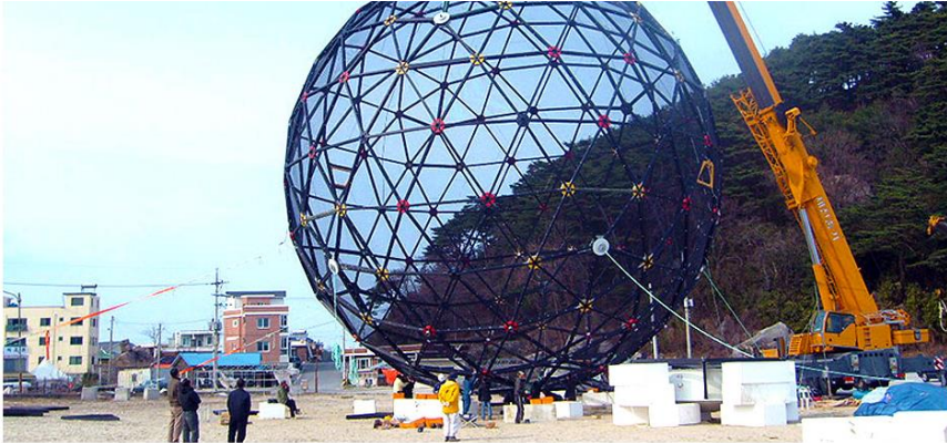
FIGURE 3: OCEAN FARM TECHNOLOGIES AQUAPOD™ NET PEN (OCEAN FARM TECHNOLOGIES, INC., 2012).
