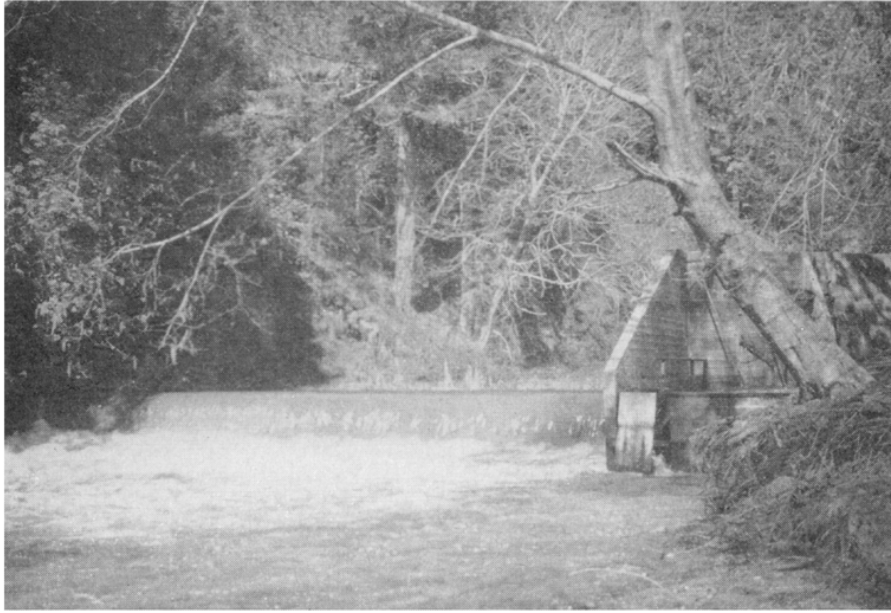
FIGURE 3. Waddell Creek dam and trap at high water; apron submerged. Photograph by Leo Shapovalov.
