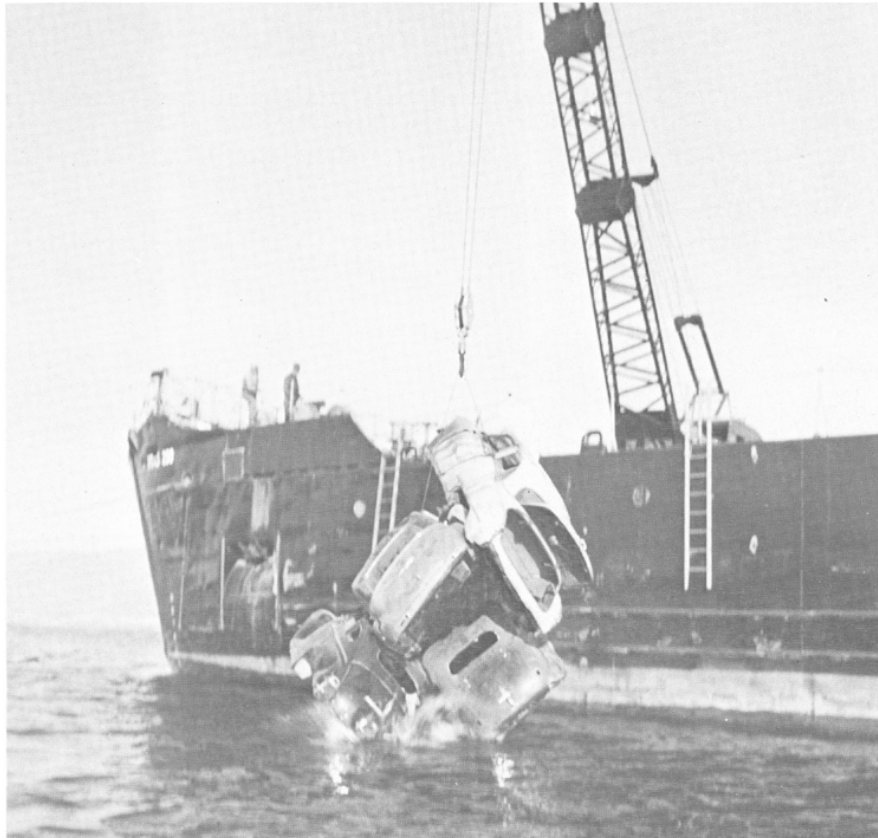
FIGURE 6 Automobile bodies, lashed together, being lowered to the sea floor, to construct a fishing reef. Photo by Charles H. Turner.
