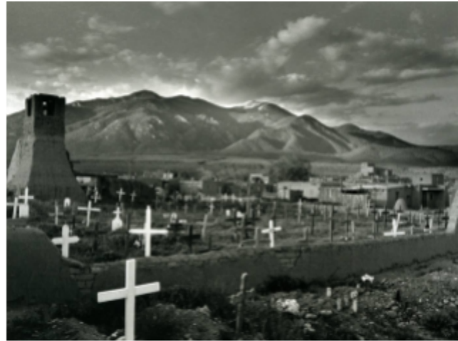
Figure 16 - 1985. The photo shows the ruins of the demolished church as a graveyard.
