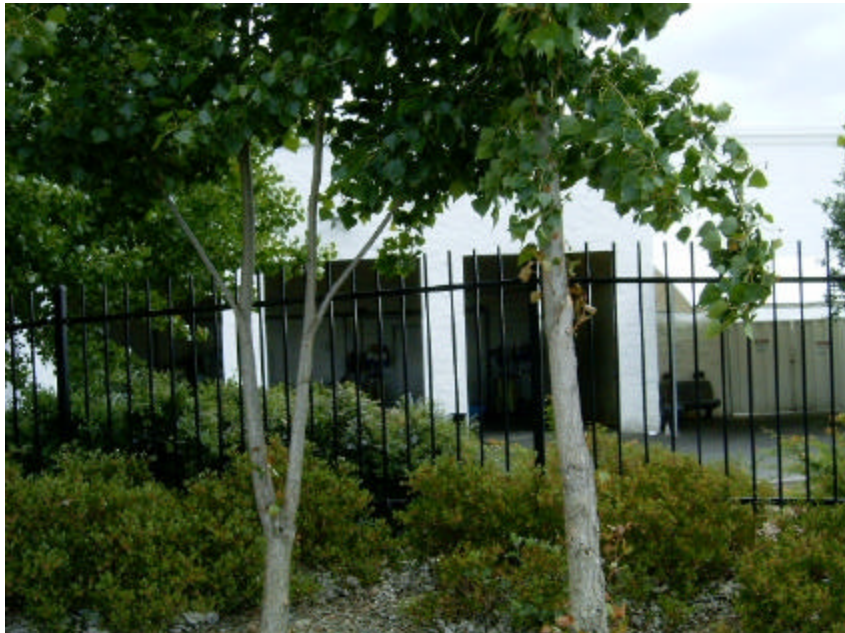
(View of garages at Buik Pontiac GMC dealership. The wall between the two garages on right was used as a benchmark for cross-section GG.)
