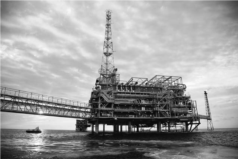
Figure 1.1. Deepwater offshore, Nigerian waters, 2006. Photo by Ed Kashi/VII. Used by permission.
