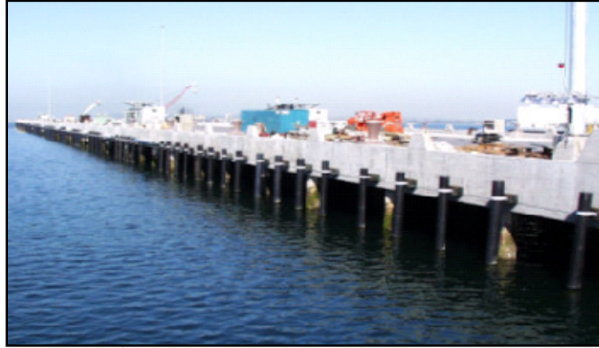
Figure (1.3): Fendering system in the U.S. Navy Pier 10, San Diego, CA
