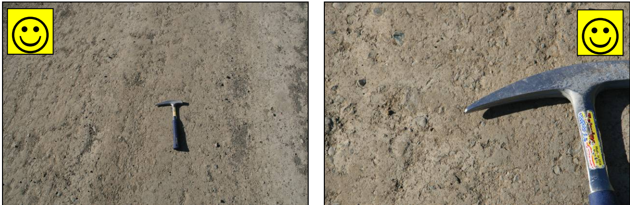
Figure 6.18: Good quality surface after final compaction.
