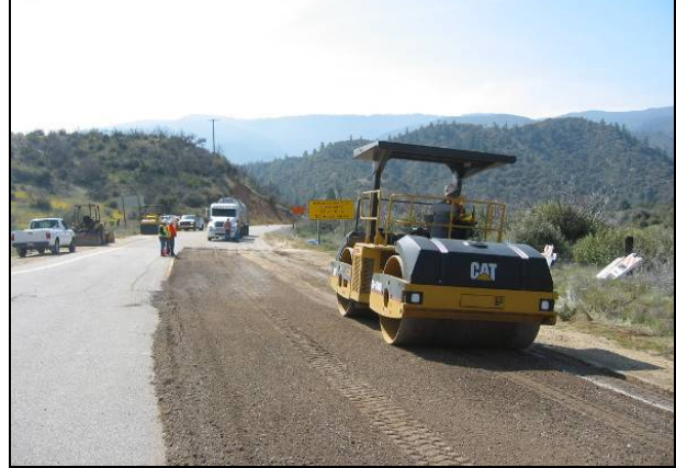
Figure 6.6: Smooth-drum roller.
