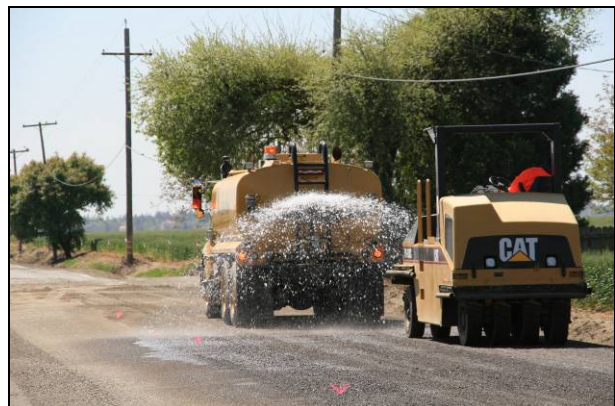
Figure 6.47: Final rolling with pneumatic-tired rollers.
