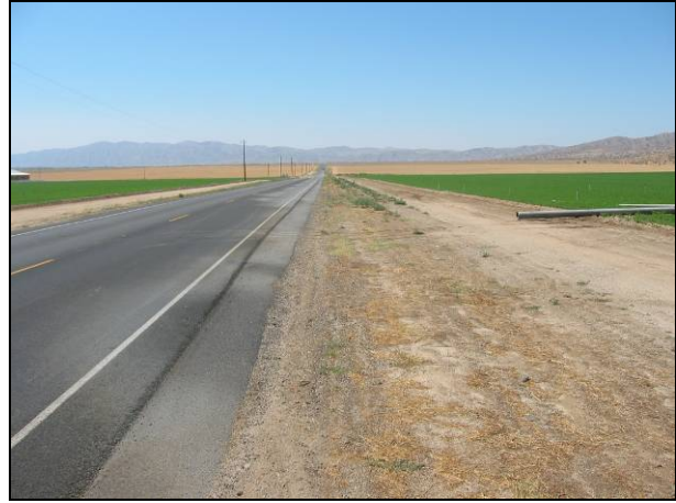
Figure 2.7: Irrigation water sprays on the road.
