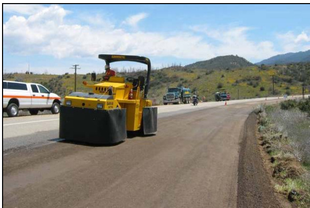
Figure 6.47: Final rolling with pneumatic-tired rollers.
