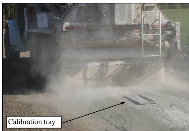
Figure 6.16: Checking active filler spread rate.
