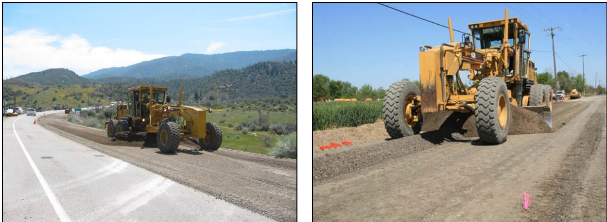
Figure 6.43: Shaping and final levels with the grader.
