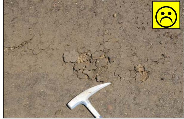
Figure 6.45: Laminations after grading.
