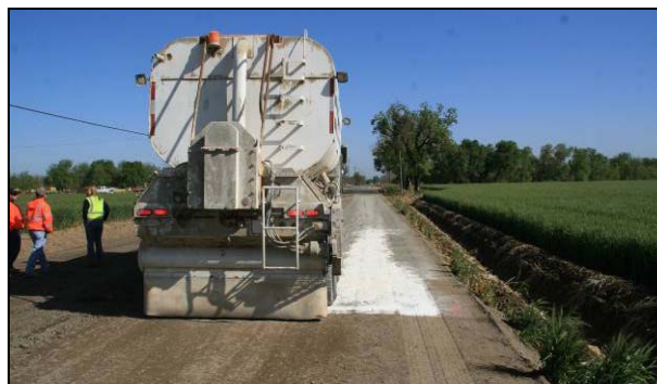
Figure 6.3: Active filler spreader.
