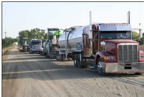
Figure 6.27: Tandem recycling train.
