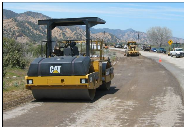
Figure 6.46: Smooth-drum roller behind grader.
