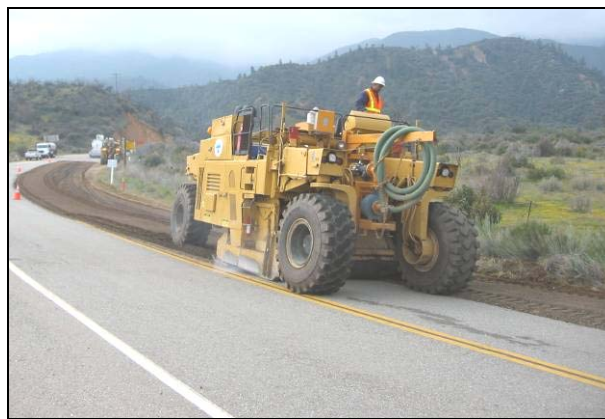
Figure 6.19: Pre-pulverization on FDR-FA project
