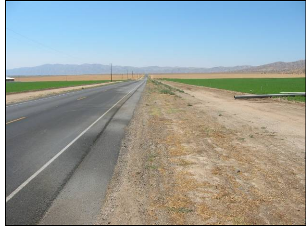
Figure 2.7: Irrigation water sprays on the road.
