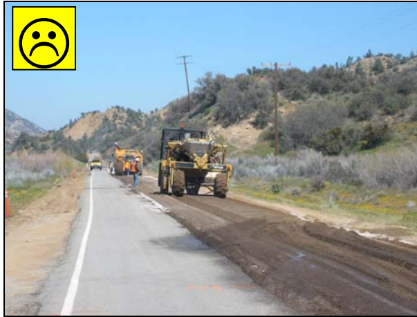
Figure 6.33: Water application between recycling train and roller before initial compaction.
