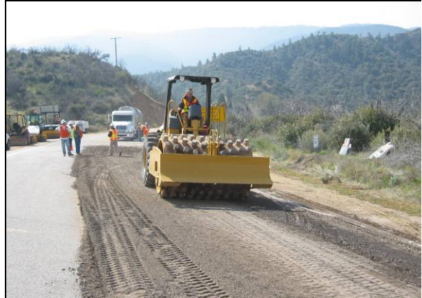
Figure 6.38: Padfoot impressions after multiple passes.
