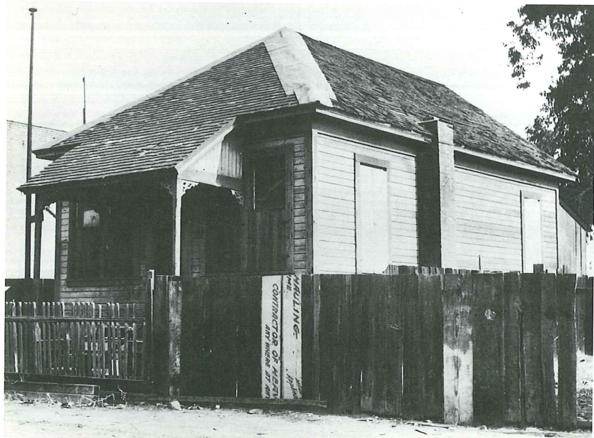
FIGURE 2.3 The Apablasa family homestead, credited as Los Angeles' oldest wooden structure, was razed as part of the Chinatown demolition. Photo courtesy of Regional History Center, University of Southern California
