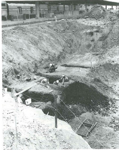
FIGURE 1.3 Excavations for the passenger bridge. Photo by R. S. Greenwood
