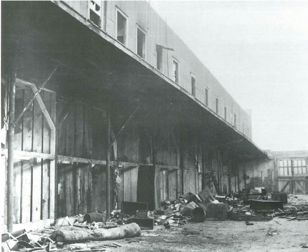
FIGURE 3.6 The location of feature 17 corresponds to the south end of the wagon shed and vegetable peddlers' storage. Photo courtesy of Regional History Center, University of Southern California, no. 8921
