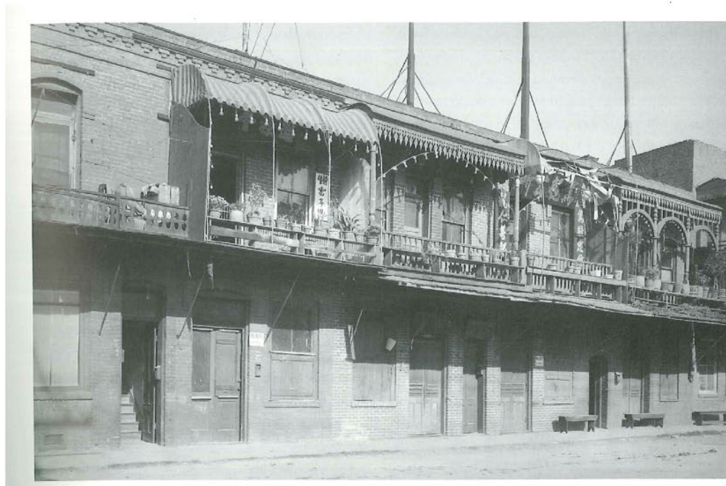
FIGURE 2.9 Wooden balconies were sometimes ornamented profusely in brilliant hues. Northern side of Apablasa Street, ca. 1933. Photo courtesy of California Historical Society, University of Southern California, Special Collections
