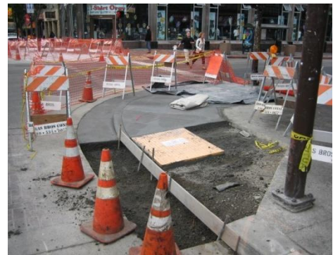
Curb ramps were installed at the corner of Telegraph Avenue and Durant Avenue.
