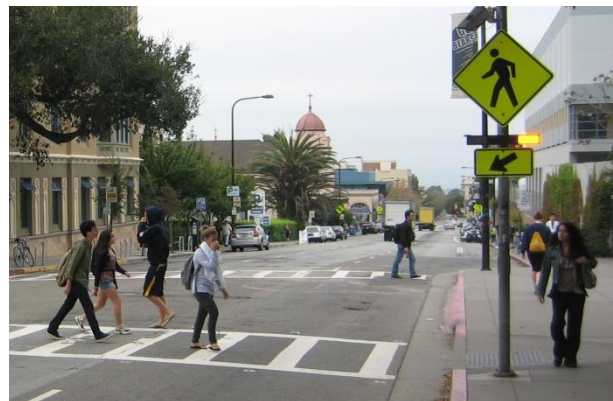
Rectangular rapid flashing beacons emphasize the pedestrian crossing of Bancroft Way at Dana Street.
