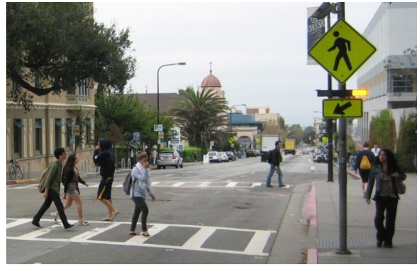
Rectangular rapid flashing beacons emphasize the pedestrian crossing of Bancroft Way at Dana Street.
