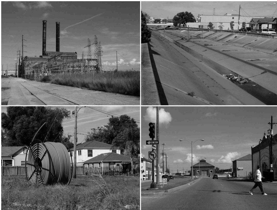
Figure 1 New Orleans infrastructure (clockwise from top left): defunct power station; high-capacity canal; pumping station; pipe awaiting placement. Photographs by author.
