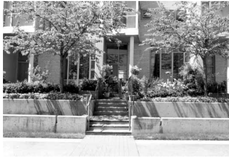
Figure 13. Typical entry terrace.
