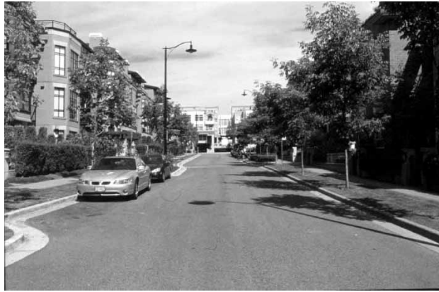
Figure 14. Typical four-storey buildings.
