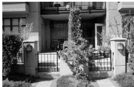
Figure 16. Typical terrace at single-level ground-floor unit.
