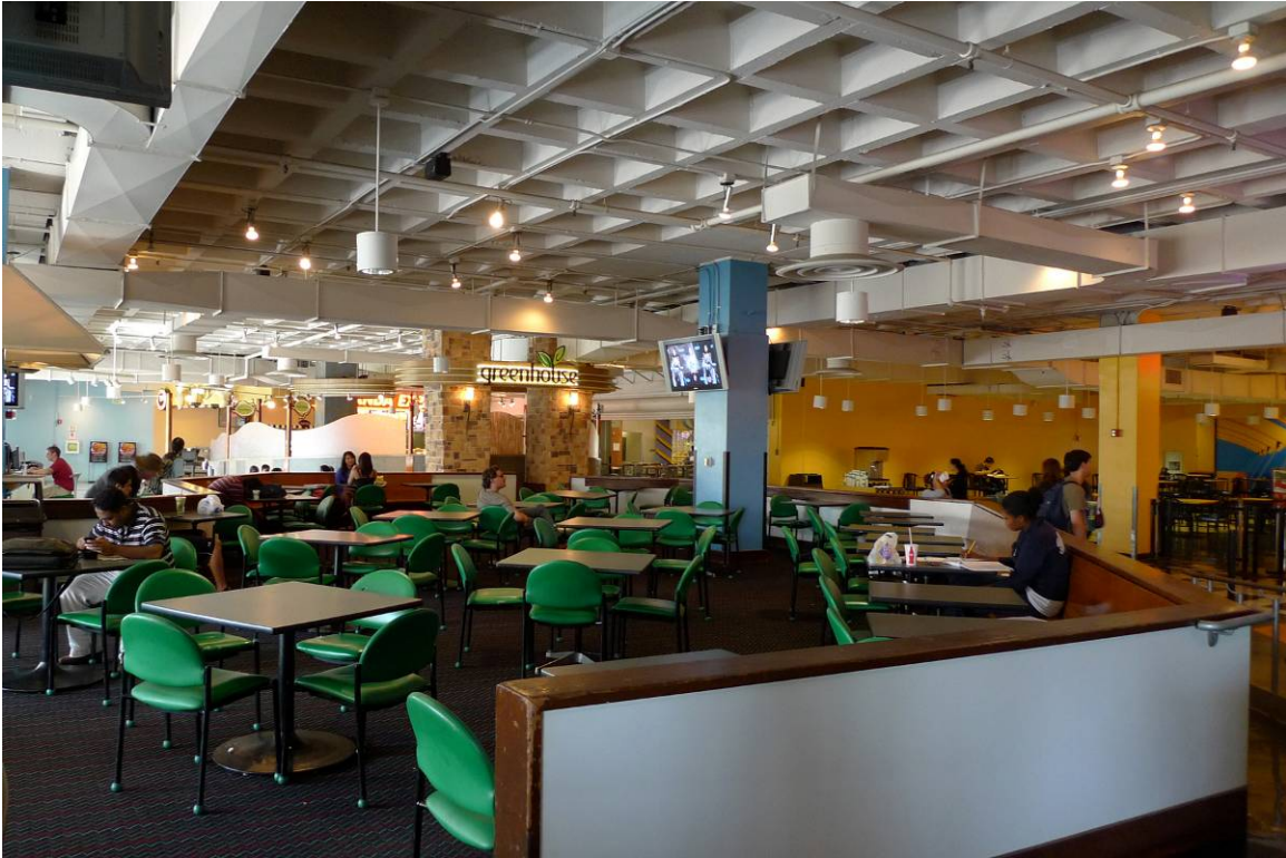
Figure 1. UCLA's dining commons in Ackerman Union. Notable updates include the walled and elevated seating area and perimeter food vendors. The original dropped ceiling has also been removed, revealing the air handling, sprinkler, and lighting systems as well as the structural waffle slab in the ceiling (photograph by author, August 2010).
