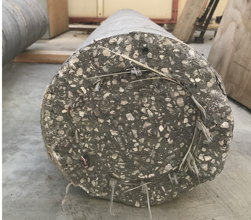
Figure 3.61: Pile 3: Cracked pile.
