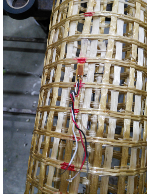
(b) Strain gauges on geogrid.
