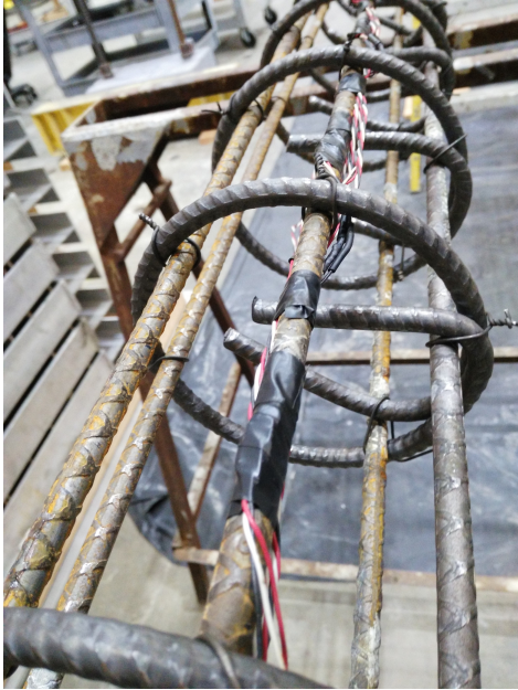
(a) Strain gauges on steel rebars.
