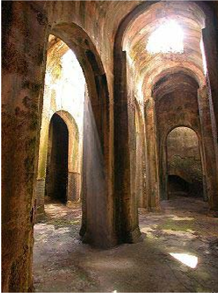
6.5a. Piscina Mirabilis at Misenum (Naples, Italy). 438
