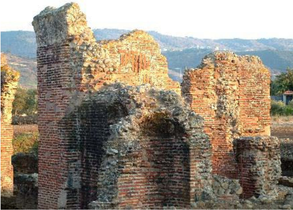
4.30. Extant structures of the private baths in Acconia di Curinga (4 th . c. AD). 186
