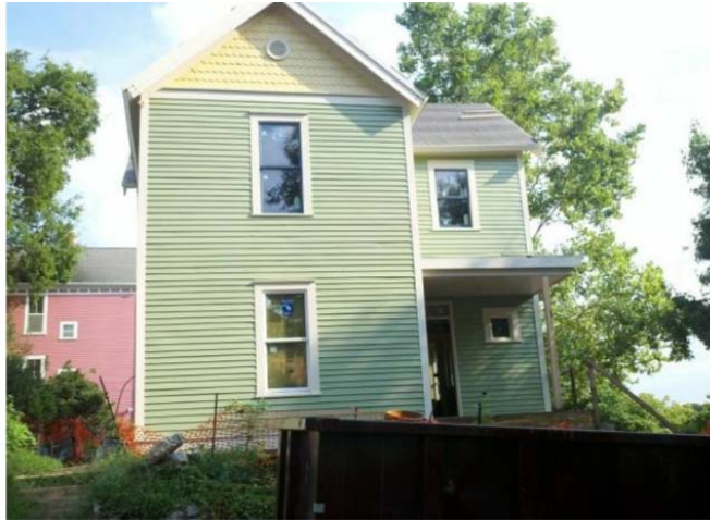
Figure 9 Front facade of the Green Home DER. Image courtesy of Oak Ridge National Lab.
