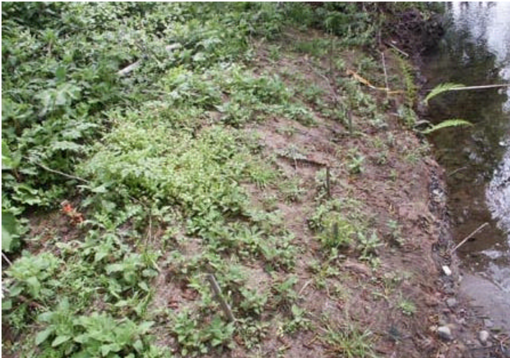
Photo 6. Riparian vegetation planted through an erosion control mat to stabilize banks.
