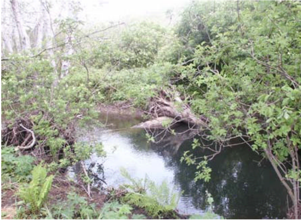
Photo 9. Pool immediately downstream of weir structure 5 (view from right bank).
