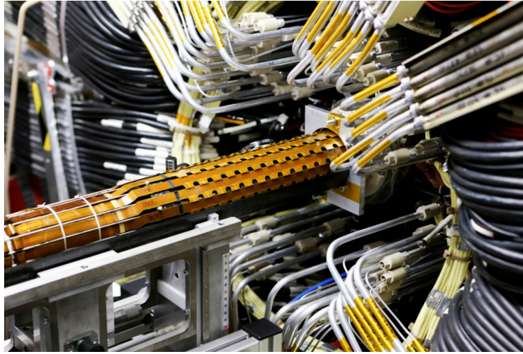
Figure 28: An image of the insertion of the IBL into the current pixel detector [27].
