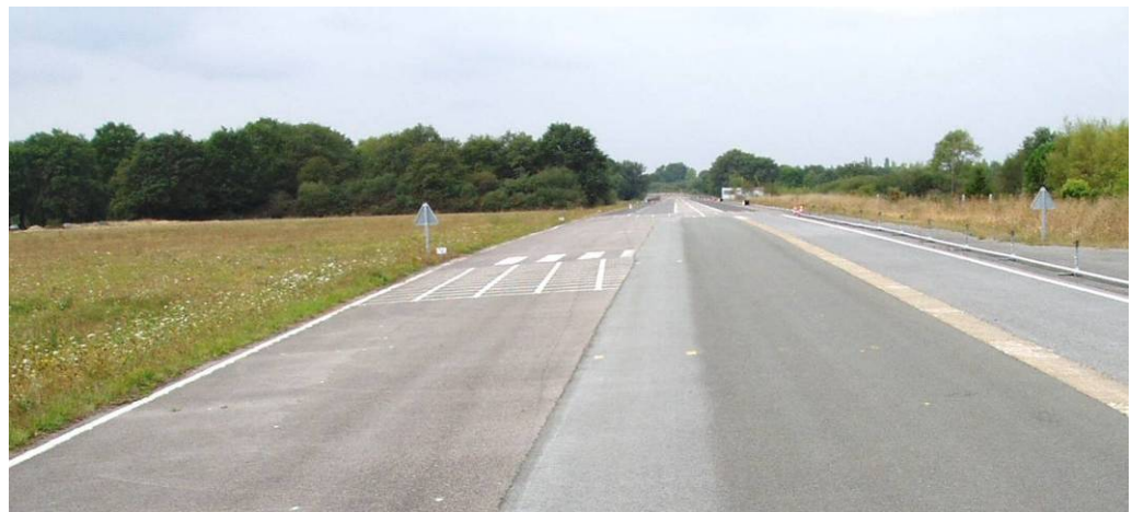
Figure 1.13. The LCPC test tracks in Nantes.
