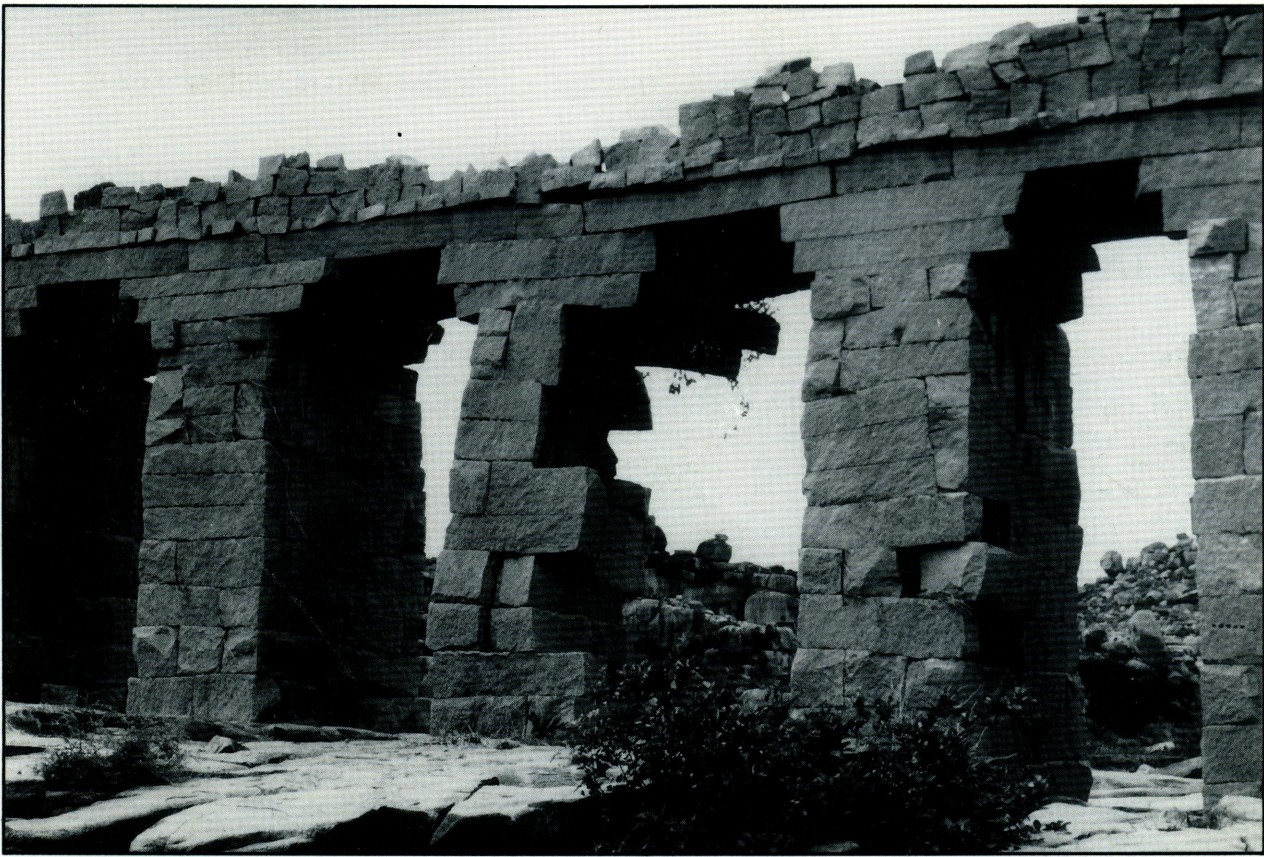
Detail of Setu aqueduct. This aqueduct carries a plastered channel that conveys water from the Anegundi Canal, north of the Tungabhadra River, to a large island just north of the village of Hampi. Individual granite blocks in the first four courses of the piers average two meters in height. Photo by K. D. Morrison.
