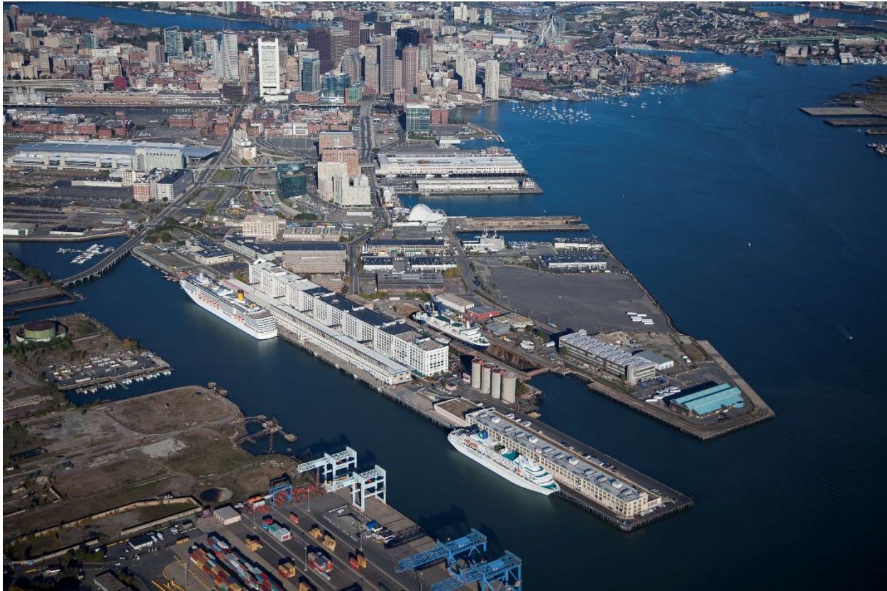
Figure 2: Aerial photography of the Marine Industrial Park
