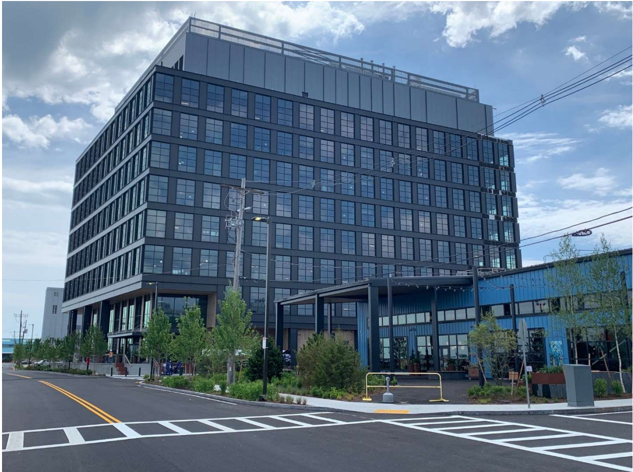
Figure 4: Picture of parcels O and P under construction
