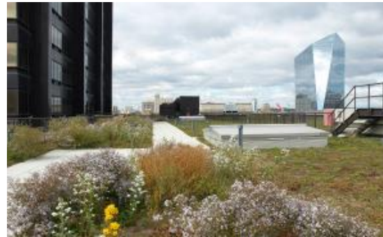
Figure 13.138 The green roof at the PECO building (Picture source: Philadelphia Water n.d.)
