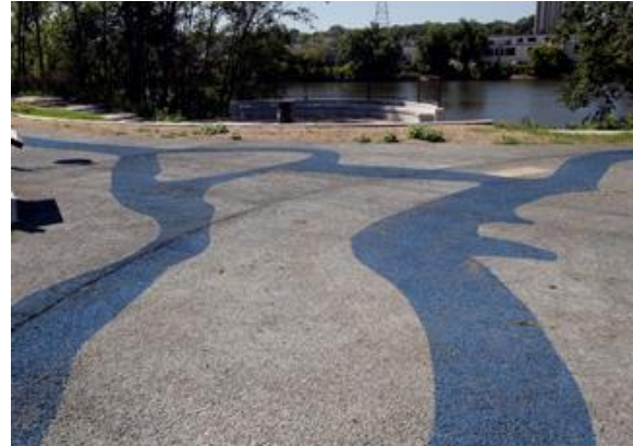
Figure 13.76 The previous concrete pavement at the Edgewater Park (Picture source: http://www.cemstone.com/contractors-project-gallery-edgewater-park.cfm , retrieved January 22, 2016)
