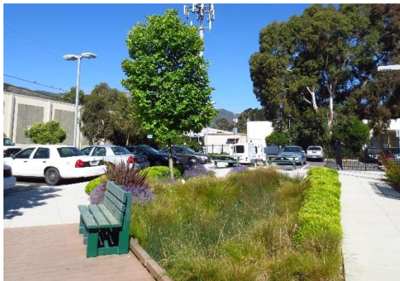
Figure 5.27 Rain garden or bioretention basin at Brisbane City Hall
