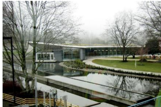
Figure 13.134 The ecorooftop at the Columbia Boulevard Wastewater Treatment Plant (Picture source: Cunningham 2014)
