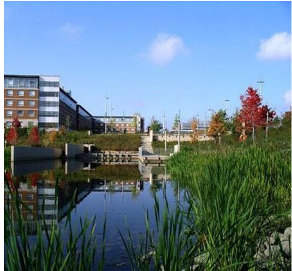
Figure 13.109 The stormwater pond at Durham College (Picture source: https://www.pinterest.com/slowottawa/urban-hydrology/ , retrieved January 22, 2016)
