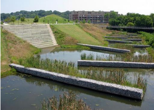
Figure 13.115 The gabion structures at Renaissance Park (Picture source: https://www.pinterest.com/yalan_12935/landscape-design-detail/ , retrieved January 22, 2016)
