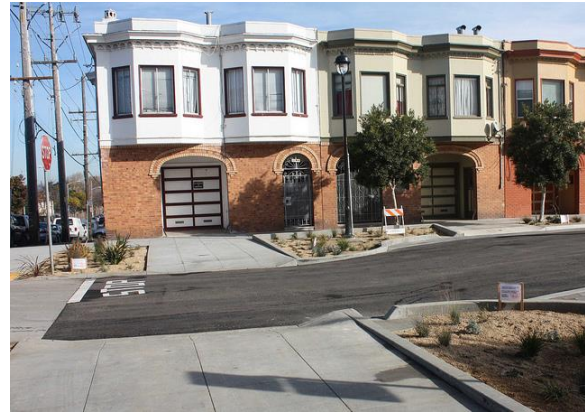
Figure 5.11 Bioretention planters at Newcomb Avenue (Picture source: http://sf.streetsblog.org/category/issues-campaigns/greenstreets-issues-campaigns-2/ , retrieved October 10, 2015)
