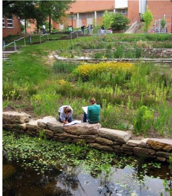
Figure 13.27 The stormwater wetland and pond at Sidwell Friends Middle School (Picture source: http://landscapeperformance.org/case-study-briefs/sidwell-friends-middle-school , retrieved January 22, 2016)
