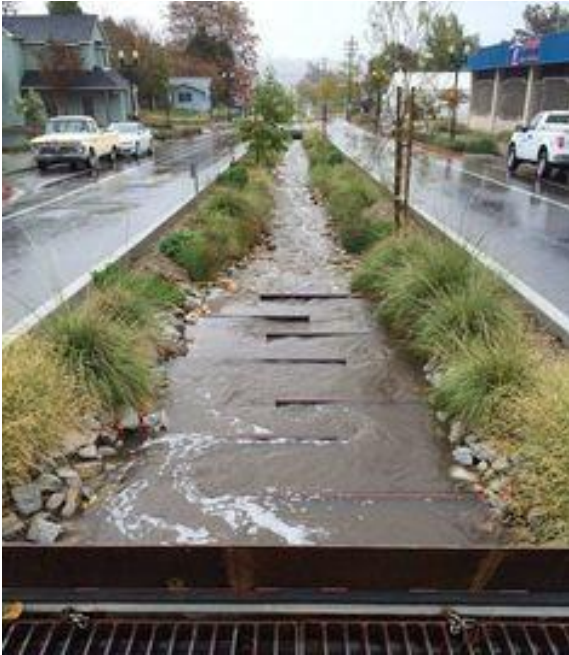
Figure 13.26 The stormwater channel at the median of 21st Street (Picture source: http://landarchs.com/award-winning-21st-street-turns-roadway-into-green-and-complete-street/ , retrieved January 22, 2016)
