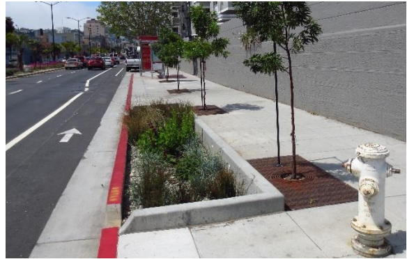
Figure 5.33-5.34 Bioretention planters at Cesar Chavez Green Street
