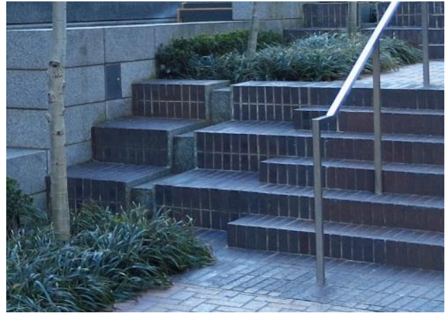
Figure 13.83 The stepped runnel at the Urban Plaza of Portland State University
