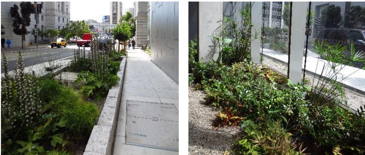
Figure 5.5-5.6 The engineered wetlands located both outside and inside the building are parts of the Living Machine at the SFPUC Headquarters
