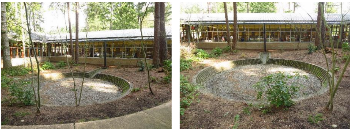
Figure 13.4-13.5 The infiltration basin at the courtyard of Maple Valley Library
