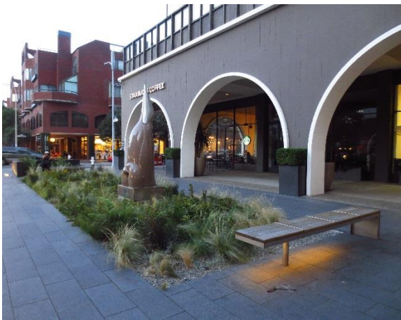
Figure 5.23 Bioretention planter and bench at Davis Court
