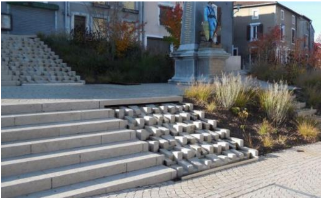
Figure 13.47 The runoff cascade in Gondrecourt-le-Chateau (Picture source: http://www.urcaue-lorraine.com/espace.php?id=23 , retrieved January 22, 2016)
