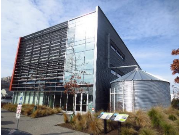
Figure 13.58 The water tank at the Center for Urban Water in Takoma
