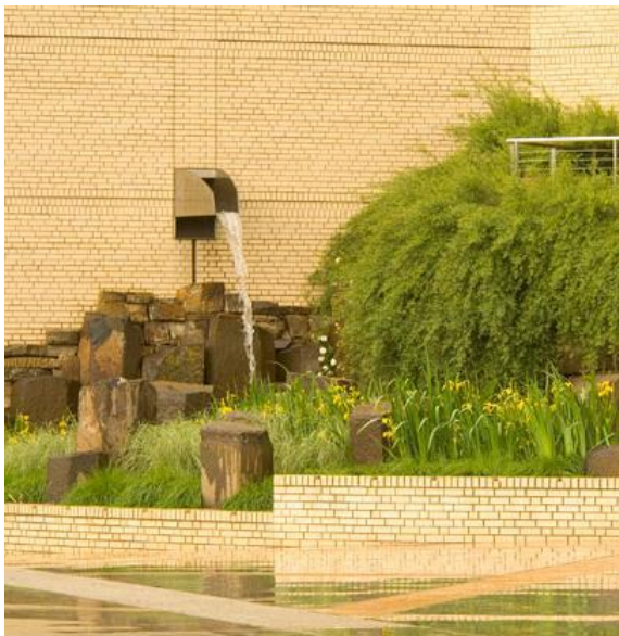
Figure 13.30-13.31 The scupper and channel at Oregon Convention Center which allow visitors to witness the story of the water's journey from rooftop to river (Picture source: https://www.asla.org/portland/site.aspx?id=43983 , retrieved January 22, 2016)
