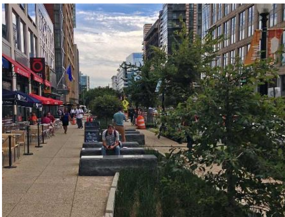
Figure 13.122 The bioretention planters along 1st Street NE in NoMa neighborhood (Picture source: http://www.nature.org/connectthedrops/protecting-the-potomac.xml , retrieved January 22, 2016)
