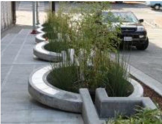
Figure 13.98 The bioretention planters at Maynard Green Street (Picture source: https://www.flickr.com/photos/rosruspix/16551474439 , retrieved January 22, 2016)
