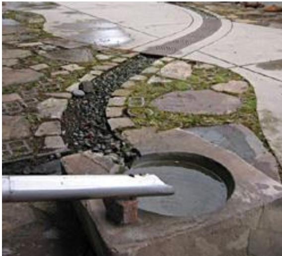
Figure 13.80 The grated channel at the courtyard of Cedar River Watershed Education Center (Picture source: https://www.asla.org/awards/2004/04winners/entry441.html , retrieved January 22, 2016)
