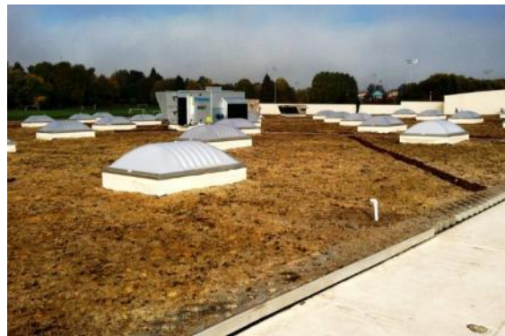
Figure 13.136 The ecorooftop at the new Walmart Portland Supercenter (Picture source: Cunningham 2014)
