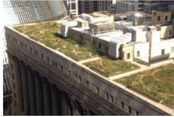
Figure 13.130 The Chicago City Hall after installing green roof (Picture source: https://www.asla.org/meetings/awards/awds02/chicagocityhall.html , retrieved January 22, 2016)
