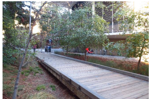
Figure 5.32 A wooden boardwalk laying over the rain garden
