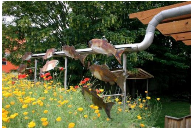
Figure 13.154 The downspout at Hawthorne Hostel (Picture source: http://www.harvestingrainwater.com/imagesvideoaudio/image-gallery/contemporary-water-harvesting-art/ , retrieved January 22, 2016)
