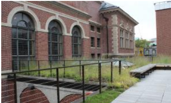
Figure 13.137 The green roof at the Law School of the University of Pennsylvania (Picture source: Philadelphia Water n.d.)
