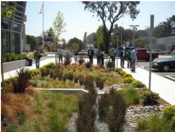
Figure 5.8 Stormwater management facility at Brisbane City Hall (Picture source: http://www.flowstobay.org/ssbrisbane , retrieved October 10, 2015)
