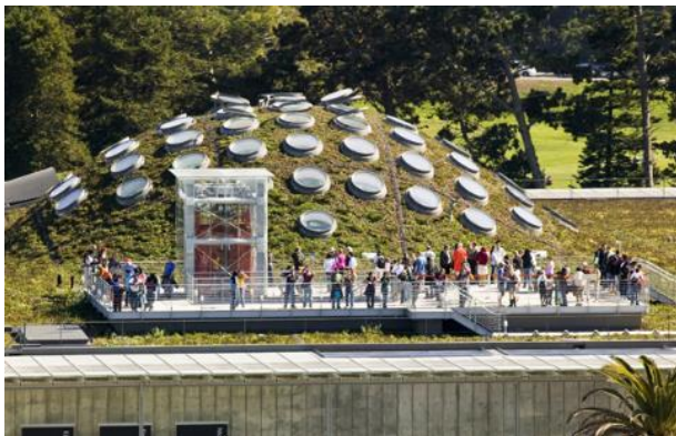
Figure 13.13 The Living Roof at the California Academy of Science which also functions as an outdoor classroom for a variety of learning activities (Picture Source: http://www.asla.org/sustainablelandscapes/cas.html , retrieved January 22, 2016)
