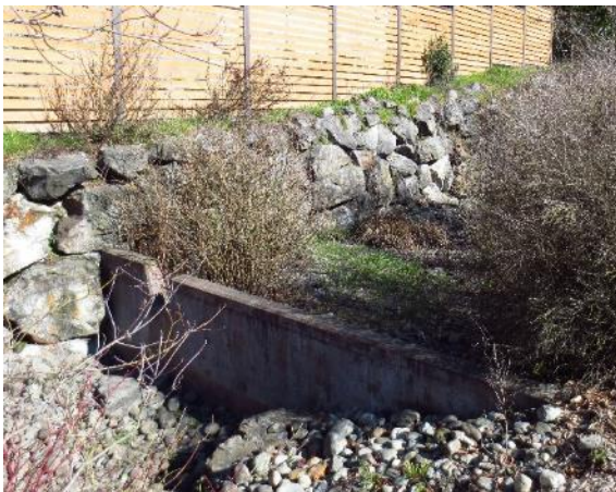
Figure 13.49 The Viewlands Cascade project in Seattle
