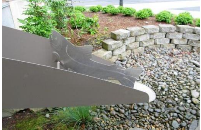
Figure 13.153 The steel salmon downspout at New Seasons Market’s Cedar Hills (Picture source: http://www.harvestingrainwater.com/imagesvideoaudio/image-gallery/contemporary-water-harvesting-art/ , retrieved January 22, 2016)
