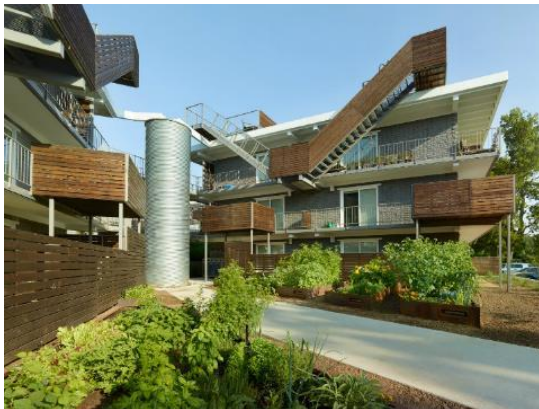
Figure 13.57 The Eco Modern Flat in Fayetteville (Picture Source: http://inhabitat.com/eco-modern-flats-renovation-is-the-first-multifamily-leed-platinum-project-in-arkansas/eco-modern-flats-modus-studios-1/ , retrieved January 22, 2016)
