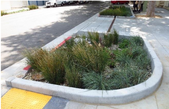
Figure 5.33-5.34 Bioretention planters at Cesar Chavez Green Street
