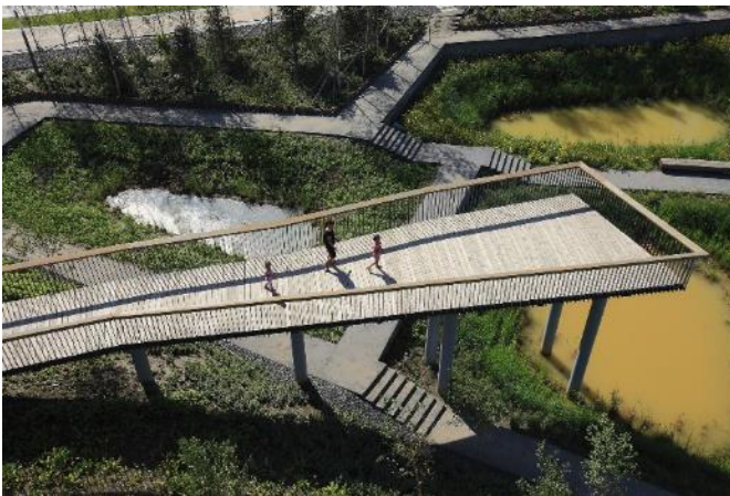
Figure 13.116 The walkway at Qunli Stormwater Park (Picture source: http://www.archdaily.com/446025/qunli-stormwater-wetland-park-turenscape , retrieved January 22, 2016)
