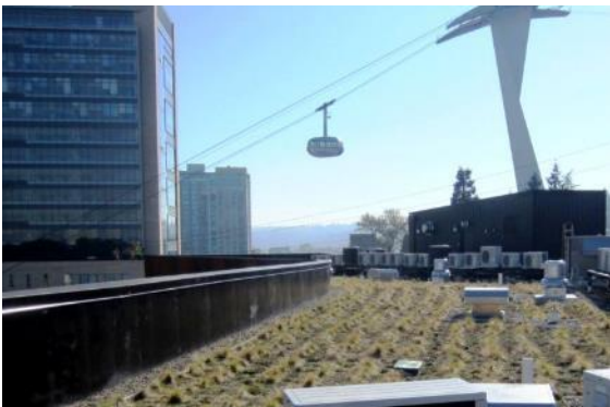
Figure 13.135 The ecorooftop at the Emery Apartments in the South Waterfront district (Picture source: Cunningham 2014)
