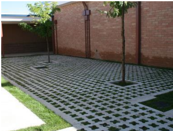
Figure 13.92 The use of grass and pavers at the New High School Campus for the Cultural Institute (Picture source: https://www.pinterest.com/patriciati/monte/urban-drainage , retrieved January 22, 2016)
