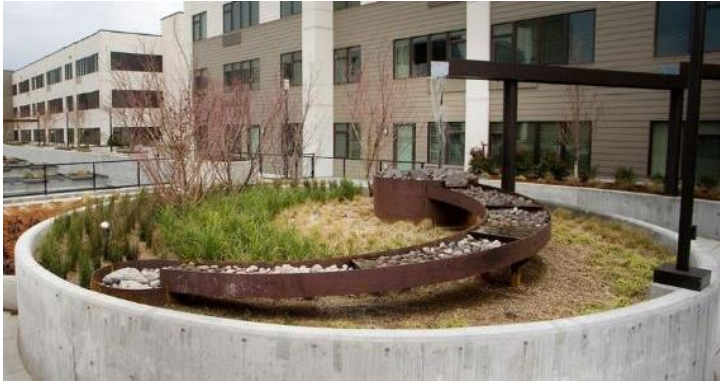
Figure 13.150 The downspout at Grant Park Village (Picture source: http://walshconstruction.co.com/our-work/grant-park-village/ , retrieved January 22, 2016)
