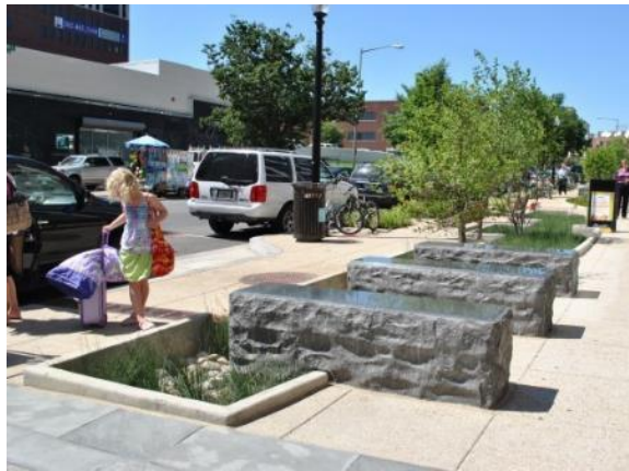
Figure 13.99 The design of bioretention planters at NoMa neighborhood (Picture source: http://parkerrodriguez.com/const2.html , retrieved January 22, 2016)
