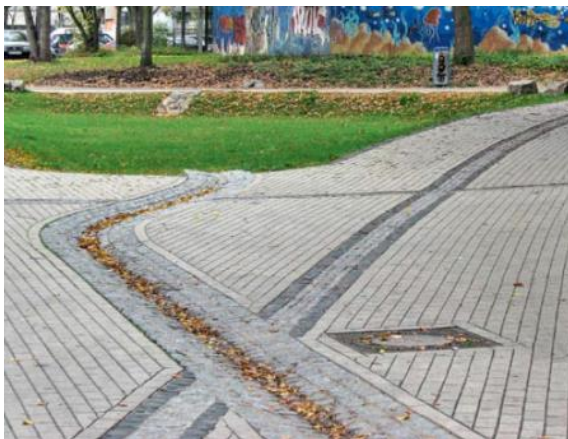
Figure 13.63 The open gutter at Scharnhorst-Ost neighborhood (Picture source: Backhaus and Fryd 2013: 55)
