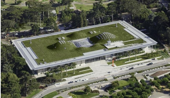
Figure 5.4 The green Living Roof located atop the California Academy of Science (Picture source: http://www.calacademy.org/our-green-building , retrieved October 10, 2015)
