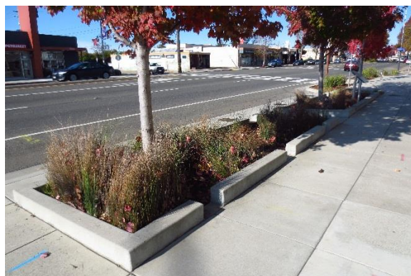
Figure 5.35 Bioretention planters at San Pablo Avenue in El Cerrito
