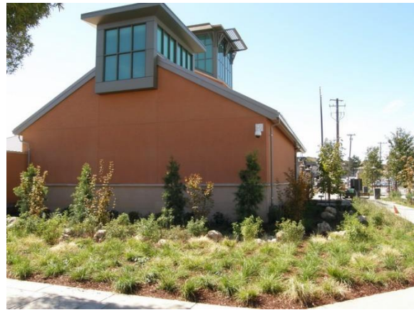
Figure 5.9 Stormwater management facility at El Cerrito City Hall (Picture source: http://bluegreenbldg.org/wp-content/uploads/2008/09/bgeccityhallbioretentionoverall.jpg , retrieved October 10, 2015)
