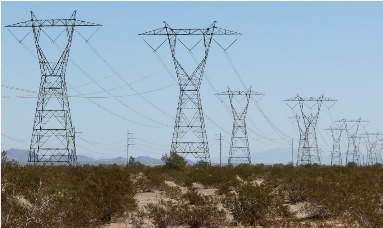
Figure 3-1. Lattice steel transmission towers in the lower Colorado Desert.
