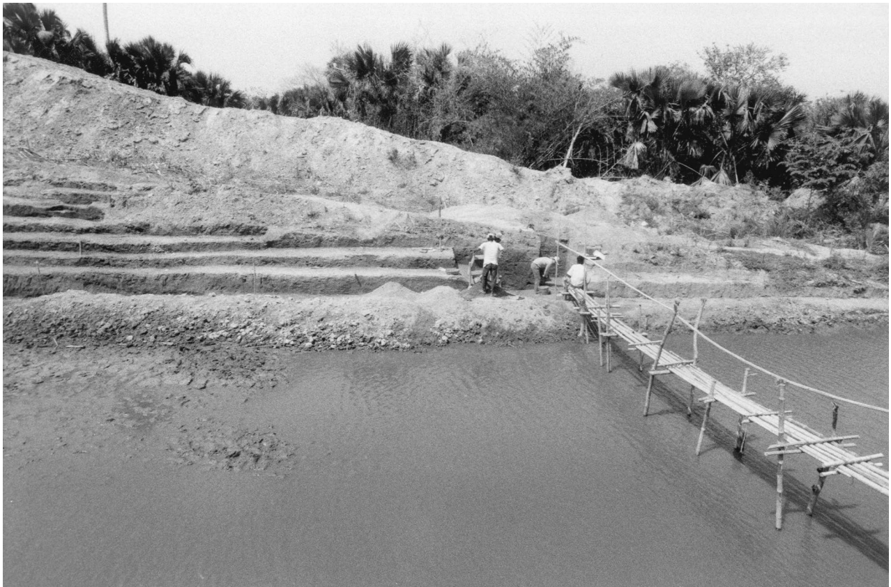
Figure 4.9. Excavations in progress in N95W0. Note again the large mass of bulldozer backdirt in the background.
