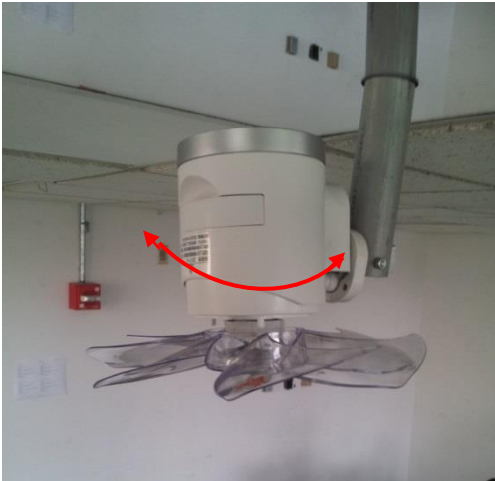
Figure 77 Toshiba floor fan mocked up in the ceiling (CBE environmental chamber)
