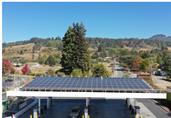
(a) 60 kW local solar power capacity
