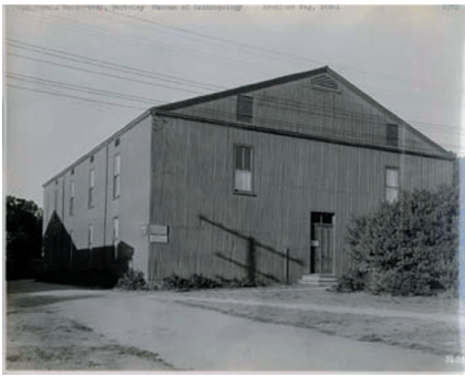
View of the “tin shack” storage structure near Faculty Glade.
