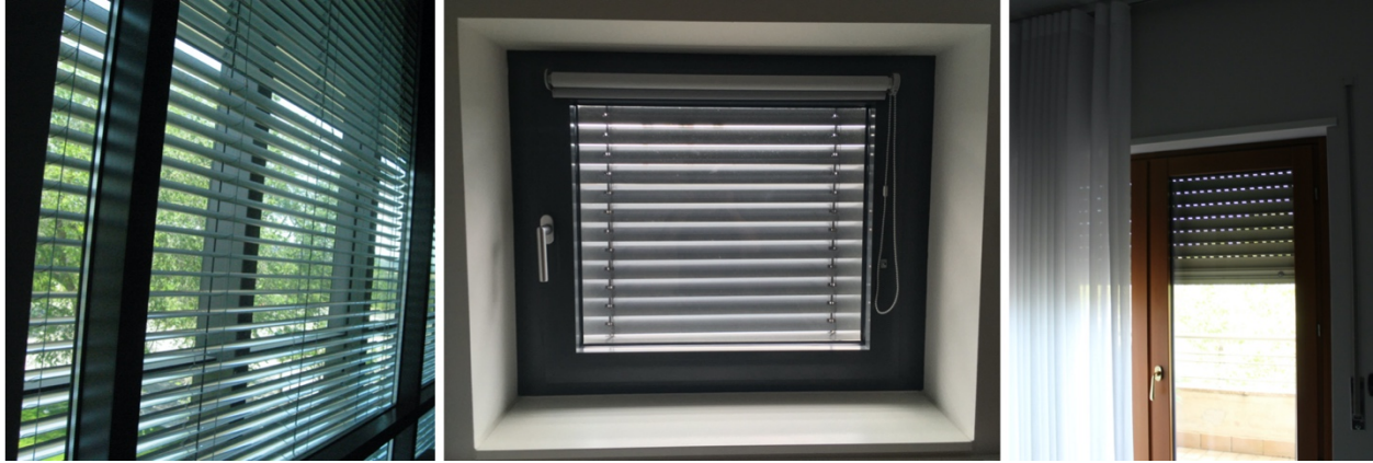
1 2 Figure 3: Different examples of window shades/blinds: Automated perforated Venetian blinds in office with automated control (and 3 manual override)(left); Residential blinds with manual control (center); Internal curtain and external roller shades in dwelling.
