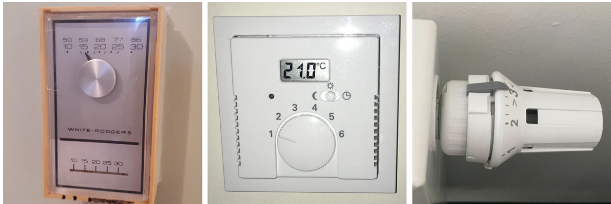
22 23 Figure 4: Examples of residential building thermostat interfaces.
