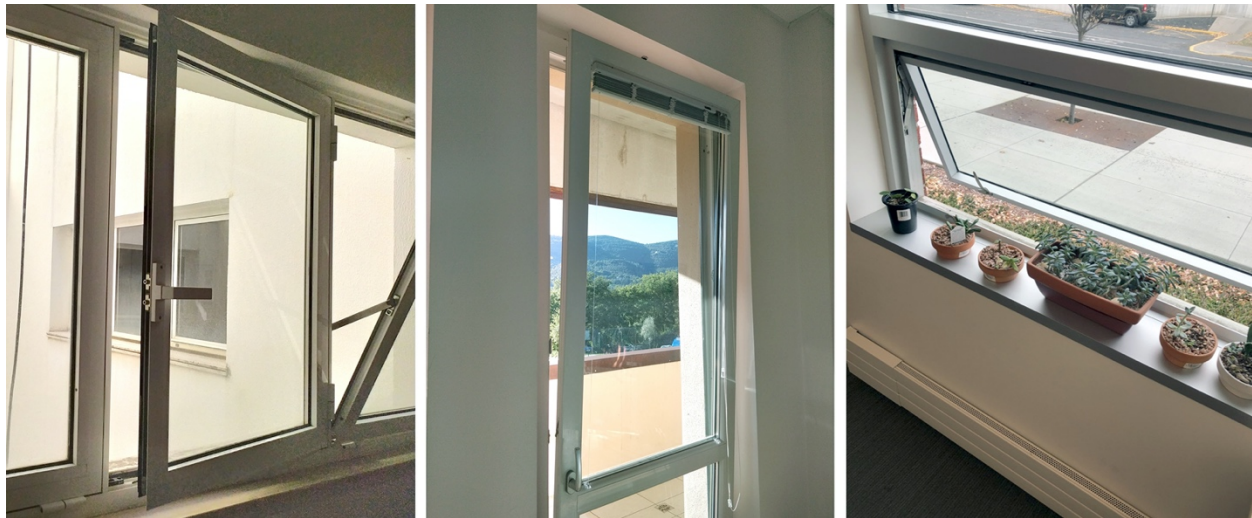
13 Figure 2: Different examples of operable windows: Single wing window with handle (left); Dual-tilt window in bottom-hung 14 configuration (center); Top-hung window (right).
