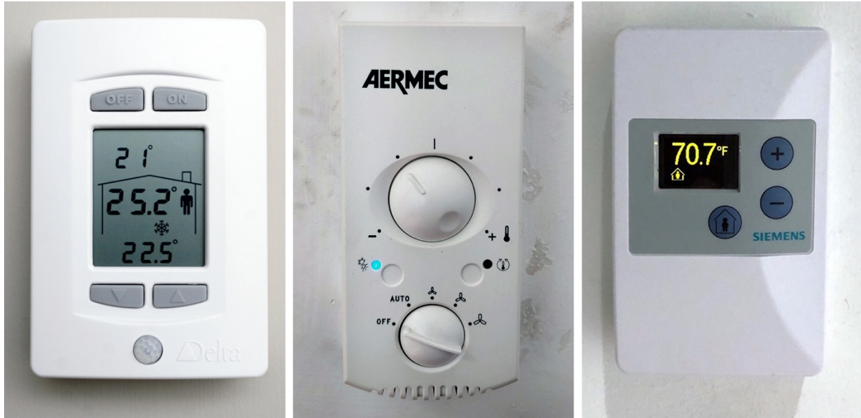
1 2 Figure 5: Examples of commercial building thermostat interfaces.
