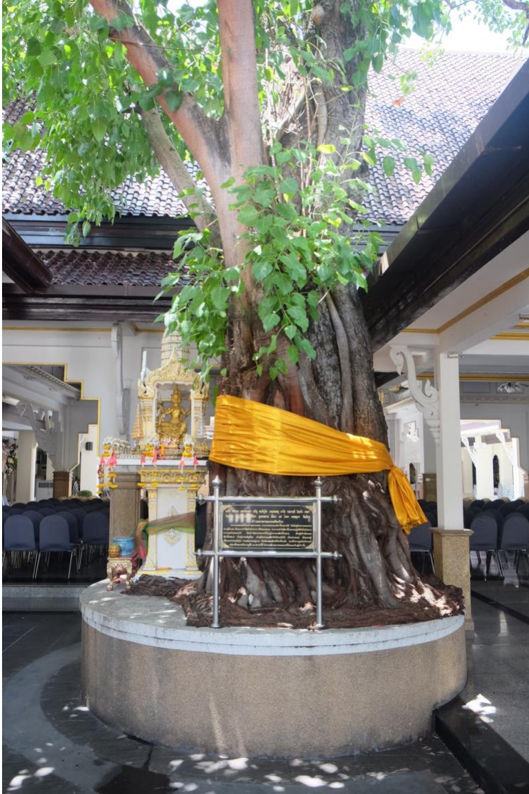
Figure 8: The Bodhi tree outgrew the concrete boulder.
