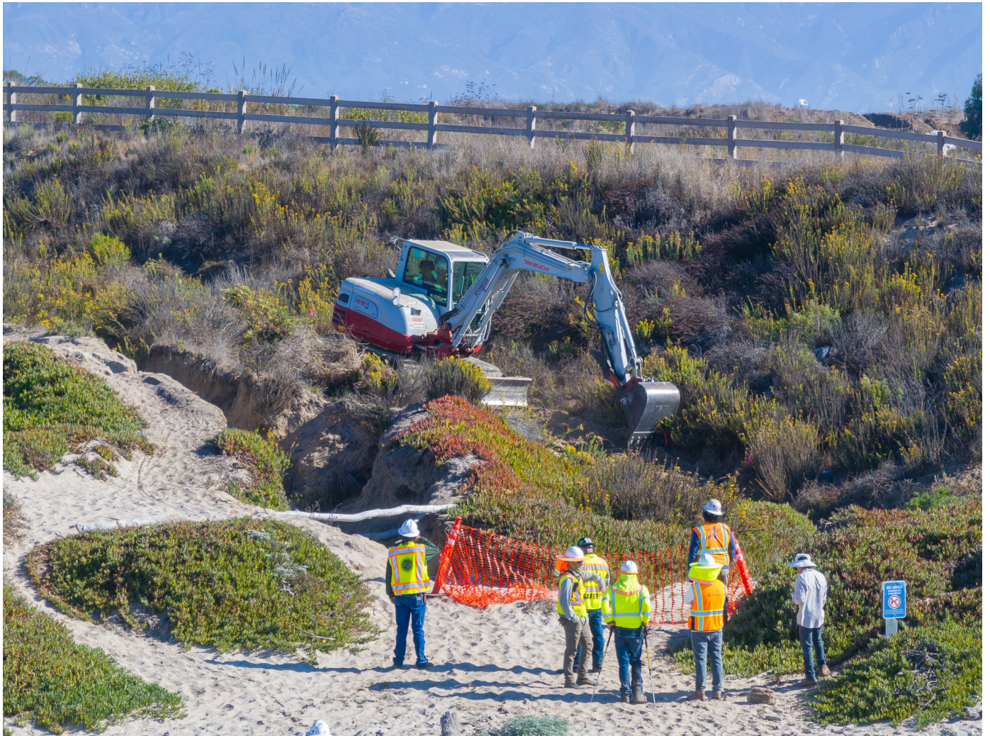
Excavation of pipeline infrastructure at COPR beach.
