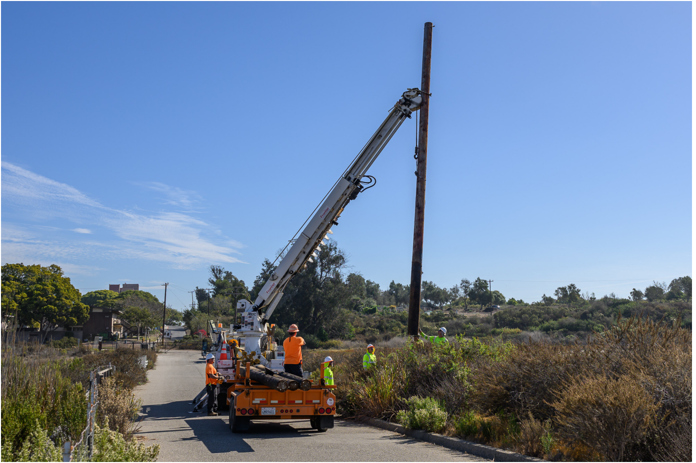
Removal of power lines on Venoco Road.
