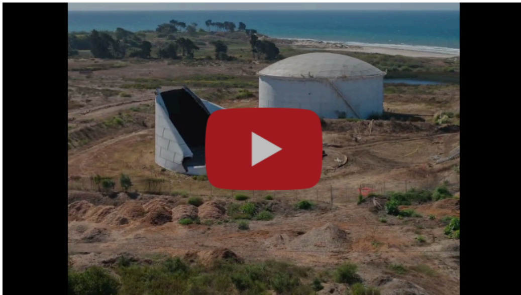
EMT Tank Demolition Timelapse - 9/20/2024.
