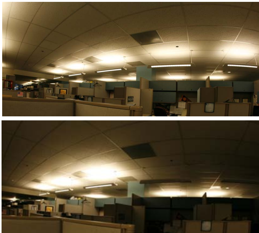
Figure 18: View of the ceiling with all nearby luminaires turned on (above) and with several luminaires turned off (below).
