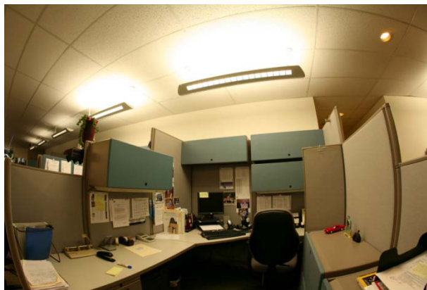
Figure 2: Cubicles lit with workstation-specific luminaires during a pilot study at the Philip Burton Federal Building.
