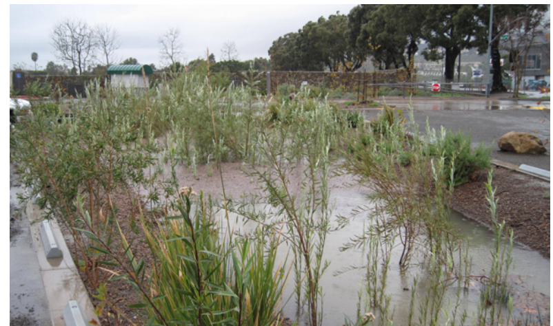
Figure 7. Runoff from surrounding areas flows into the rain garden basin, inundating the plants in this public landscape and parking area. Source: M. Myers
