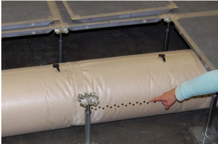
Figure 4-1 Orifices along the duct
