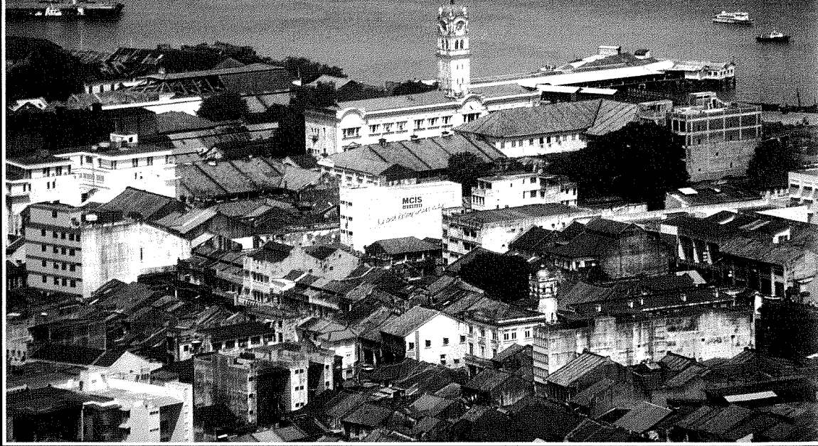
A typical roovescape in the shophouse district of Penang.
