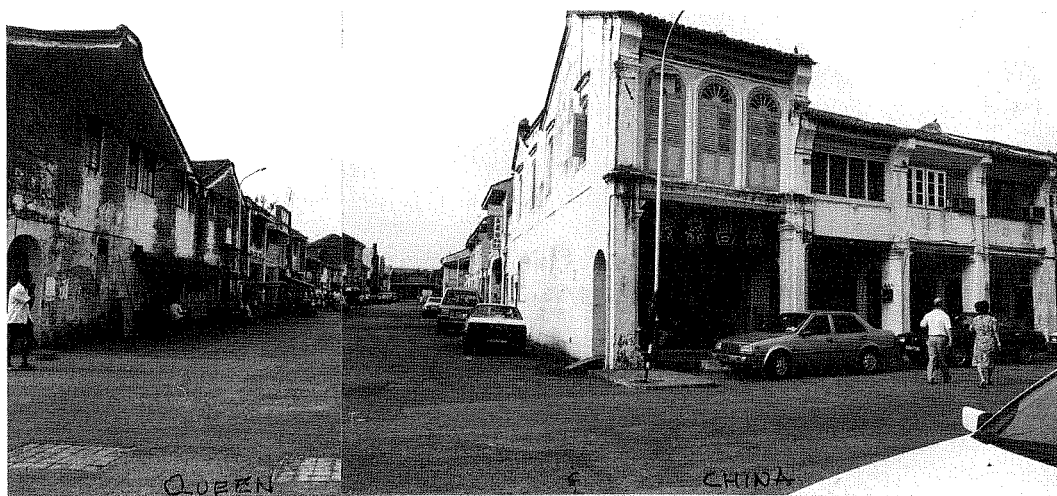
Two of the streets laid out by Francis Light. The depth of the shophouses allows for a series of light wells and courtyards.
