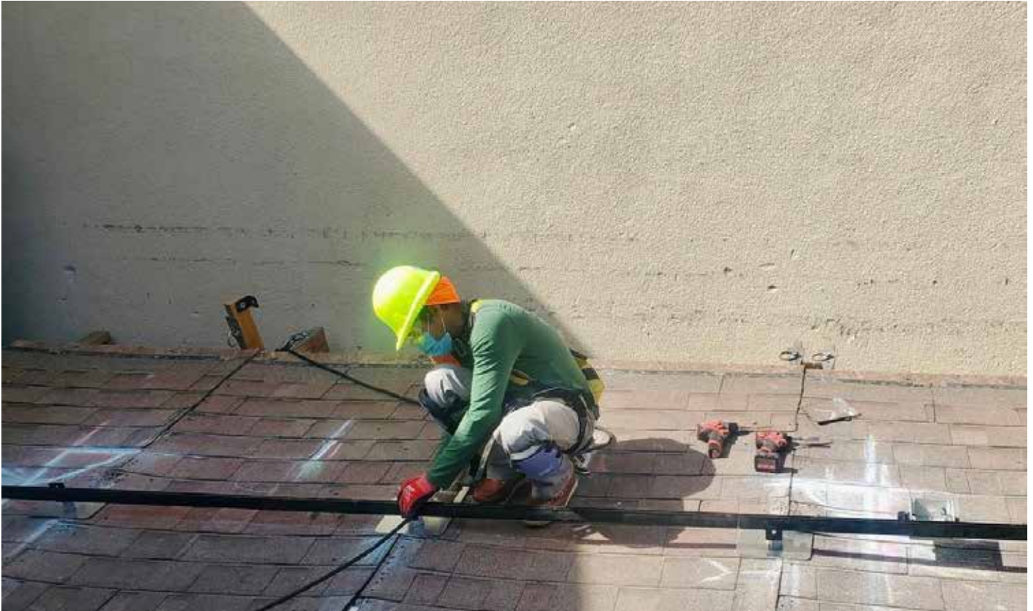
GRID Alternatives solar installation trainee. Photo credit: GRID Los Angeles
