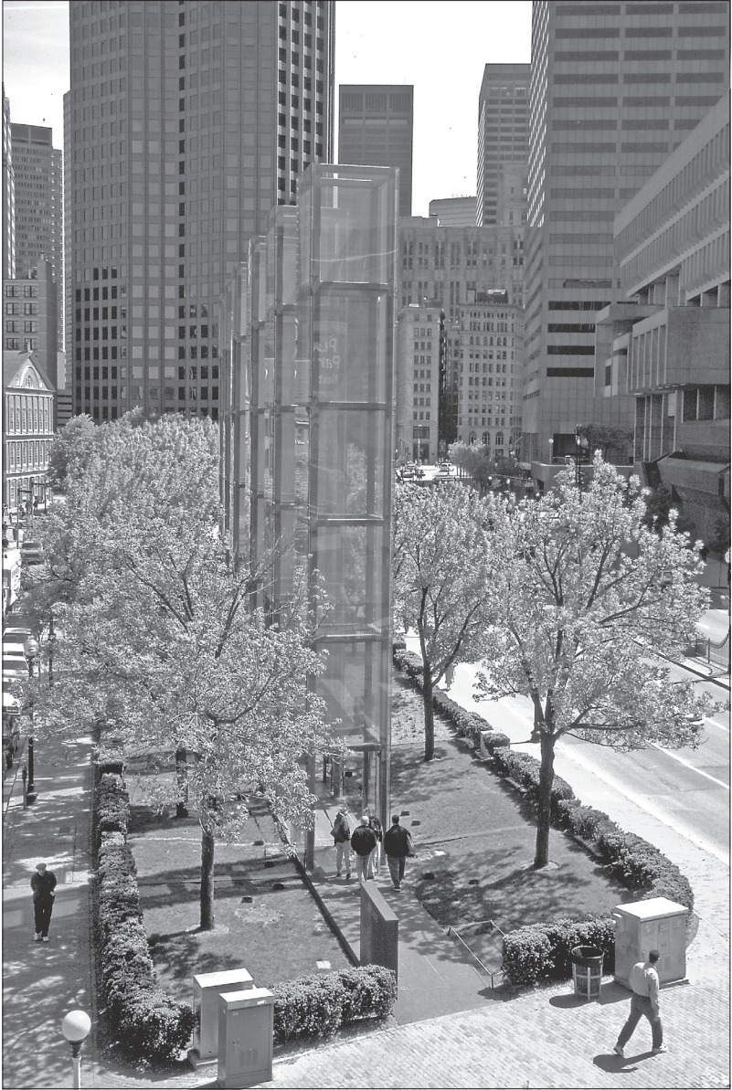
New England Holocaust Memorial, Boston (completed)
