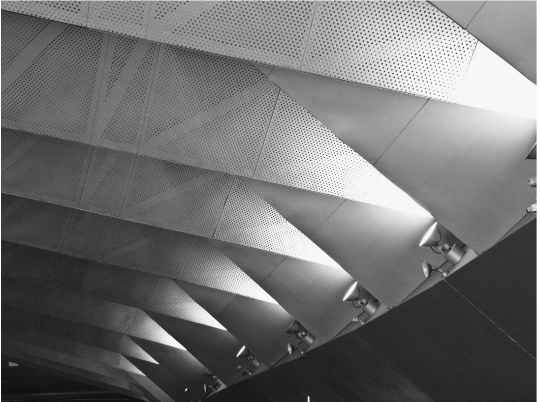
FIGURE 3.3. Interior girders at Yokohama Port Terminal, Yokohama, Japan. Building designed by Foreign Office Architects (Farshid Moussavi and Alejandro Zaera-Polo), 1995–2002. Photograph by blanco teko (CC by NC 2.0). The unique girder structure of the ceiling, covered with panels here, was likely “evolved” using genetic algorithms.
