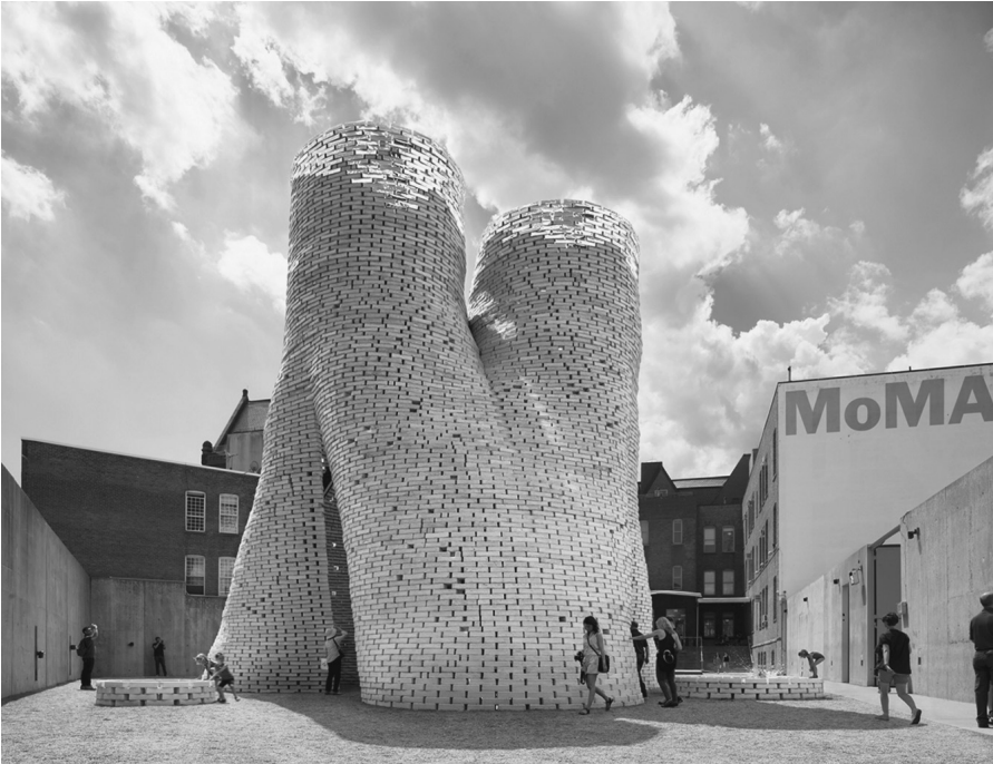
FIGURE I.3. Hy-Fi , by David Benjamin / The Living with Ecovative, 2014. Winner of MoMA PS-1 Young Architects Program, 2014. The bricks in this structure are created out of mushroom mycelium and corn stalks.
