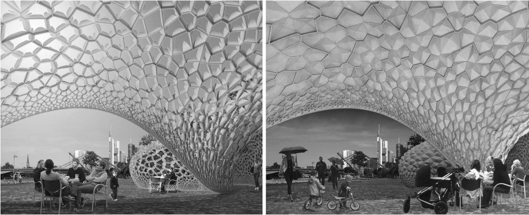
FIGURE 1.9. FAZ Pavilion, by Achim Menges, Steffen Reichert, and Scheffler + Partner, Frankfurt, Germany, 2010. The honey-combed panels of this thin plywood pavilion passively open and close in response to humidity levels in the environment, owing to the hygroscopic properties of wood.
