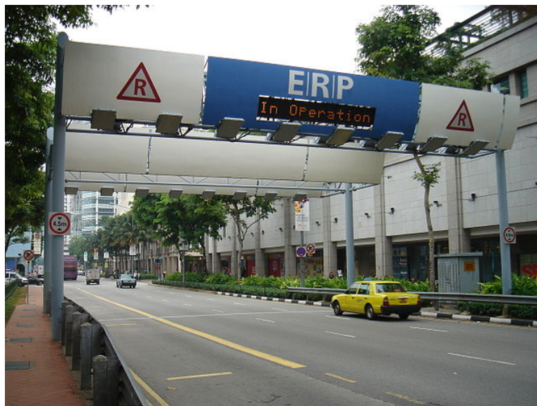
Figure 2.2: ERP gantry (Land Transport Authority, 2016)
