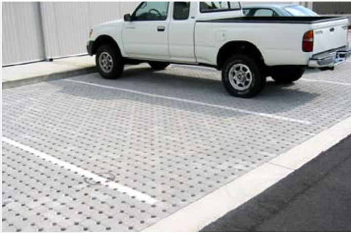
Figure 31. Permeable paving blocks reduce the impervious surface area in this parking lot. Photo: Eban Bean.
