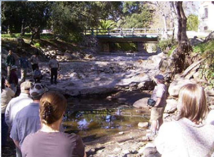
Figure 16. Intermittent section of Mission Creek in Oak Park in Santa Barbara. The stream bed has been hardened with concrete downstream of the bridge. During the dry season this prevents groundwater from replenishing the flow, while during the wet season it causes the stream to erode and undercut downstream of the concrete. The stream banks in the reach upstream of the bridge have been lined with concrete to protect the foundations of streamside buildings. Photo: L. Thompson.
