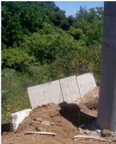
Figure 23. This barrier was placed to prevent sedimentation during road construction. Photo: S. Kocher.
