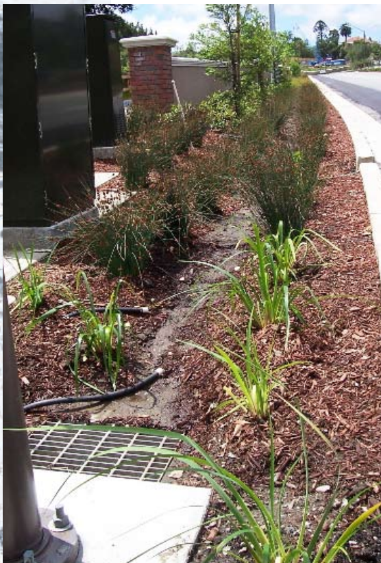
Figure 35. This bioswale was installed during a road widening project in Menlo Park, California, to mitigate for the additional runoff caused by additional impervious surfaces. The swale is constructed with a layer of aggregate under the soil and is planted with wetland species. The curb along the road has gaps to allow water to flow into the swale. A catchment was installed (under the grate) to allow sediment to settle out of the storm water before discharge to the creek. Photo: R. Harris.
