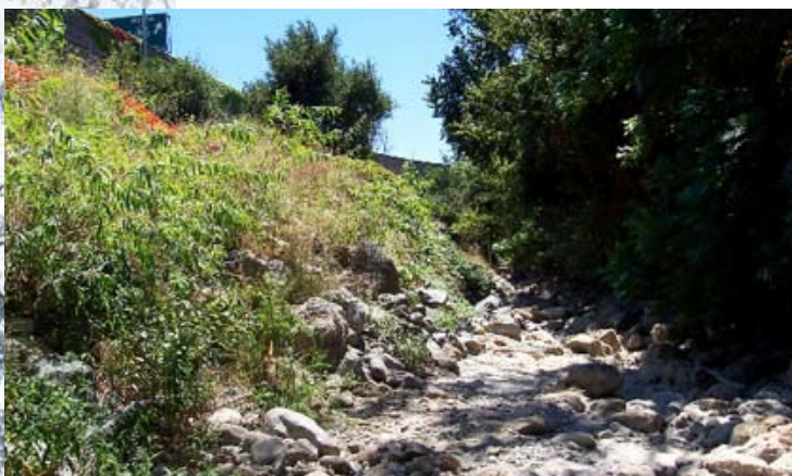
Figure 22. This stream bank stabilization project involved excavating an unstable stream bank and stabilizing it with a bioengineered structure that incorporates riparian vegetation. Photo: R. Harris.
