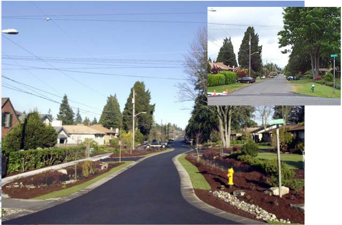
Figure 29. Seattle's Street Edge Alternatives project involved calming traffic by narrowing and curving the roadway and installing storm water retention swales. (Inset: street before the project.) Source: © 2005, Seattle Public Utilities, used with permission.
