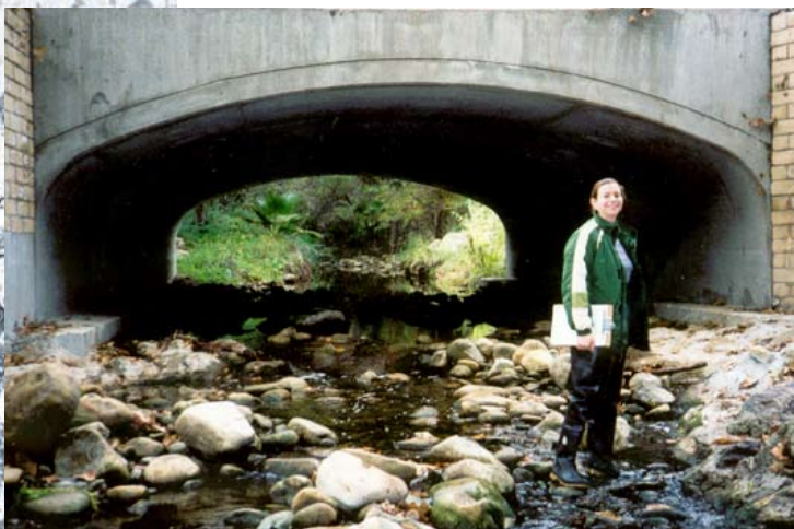
Figure 19. Prefabricated bridge crossing on a coastal stream in Ventura County, California. Photo: L. Thompson.
