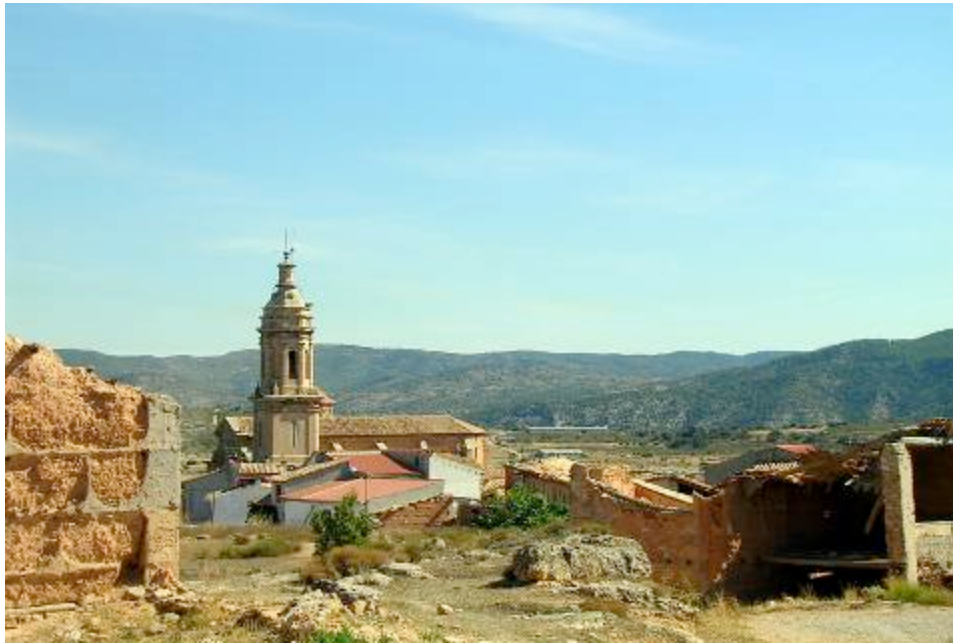
Appendix Photo 3: Abandoned structures in Aguaviva
