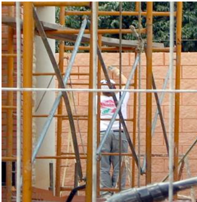
Appendix Photo 7: Aguaviva's construction industry (worker is a Romanian migrant)
