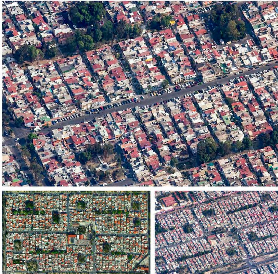
Fig. 5. Bounded grid, disrupted. In laying out the Colonia CTM Aragón, planners played with the grid form by breaking it up. Financed by the Confederation of Mexican Workers (CTM), the colonia reveals several design features unusual for Mexico City. A series of 16 linear and square green spaces ensure that most households have one within short distance. Residential stock is comprised predominantly of single-family townhouses rising two stories on modest footprints, with the space normally allotted to courtyards redistributed to the various green spaces. The central module contains a church, market, and schools. Streets afford limited ingress, and there is no way to traverse the colonia in an automobile. More unusual is the neighborhood's interior parking system, with vehicles restricted to designated thoroughfares, and many houses only accessible via narrow pedestrian walkways. These various features are reminiscent of the 'New Town in the City' planning approach of the 1960s and 1970s. While manifestly a grid, the urban morphology of the neighborhood also has a diagrammatic quality to it (see Figure 6 below).
