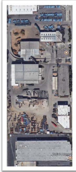
Figure 41. The industrial facility of the C&I Sector [40]
