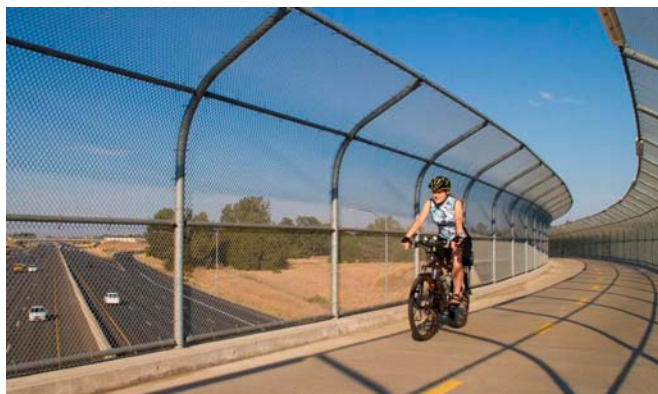
Figure B-6. Highway 50 overcrossing
