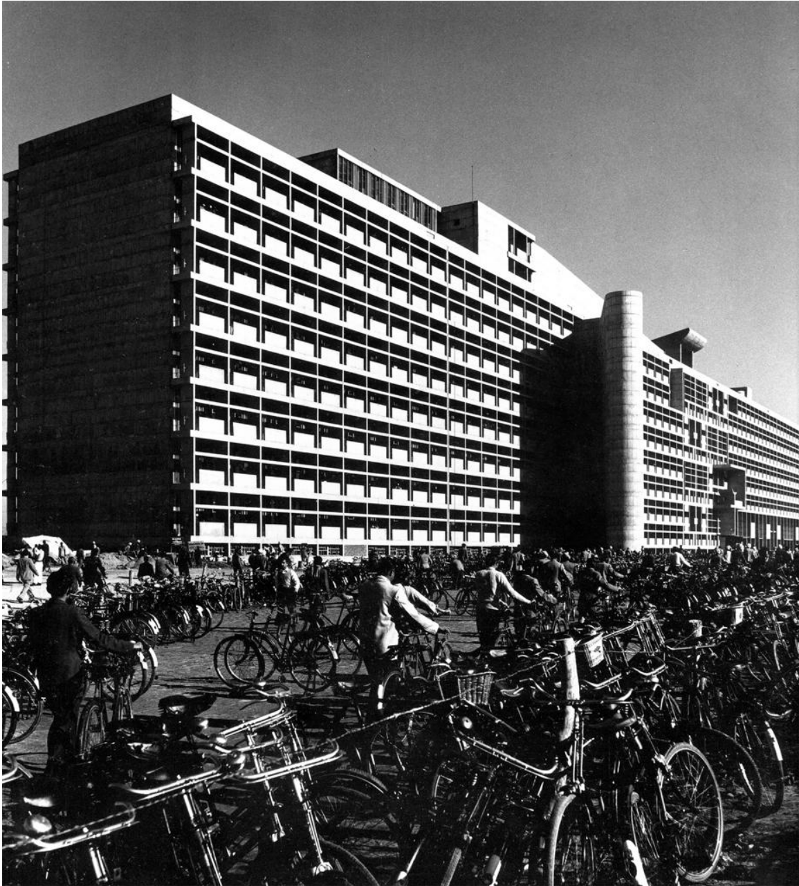
Figure 3.18. Le Corbusier, Secretariat , Capitol Complex, Chandigarh, India, c. 1951-58. Avery/GSAPP Architectural Plans and Sections, Columbia University. Retrieved from ARTstor, http://library.artstor.org/asset/AWSS35953_35953_34611298 .
