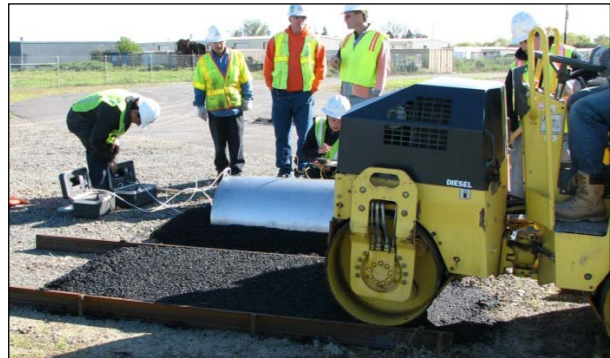
Figure 3.5: Test section compacting prior to sampling.
